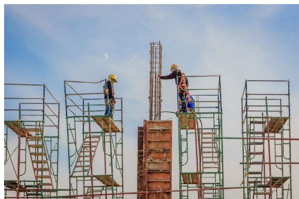
Fig. 6.1.4 Coordination during Construction Work
