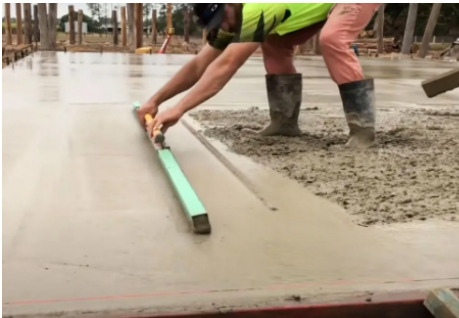
Fig. 4.2.9 Concrete Screeding
