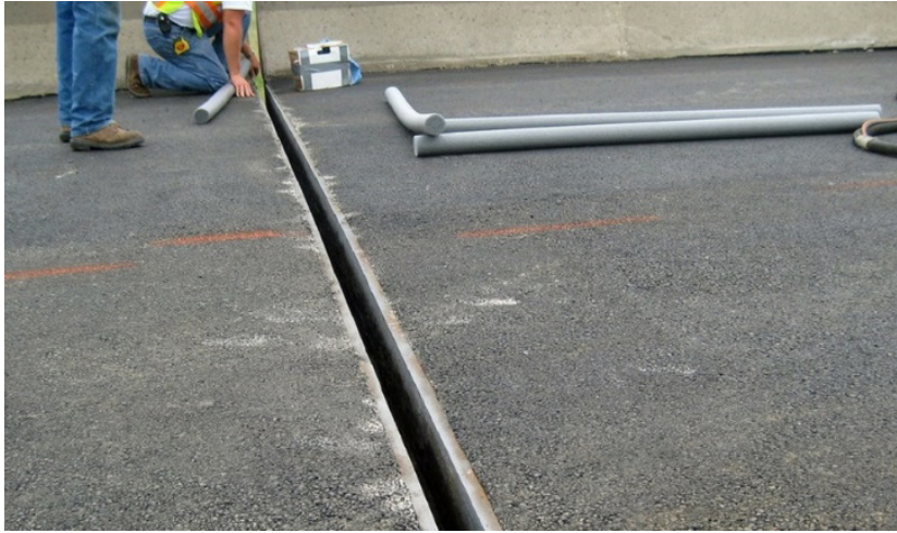
Fig.3.1.10 Expansion Joints
