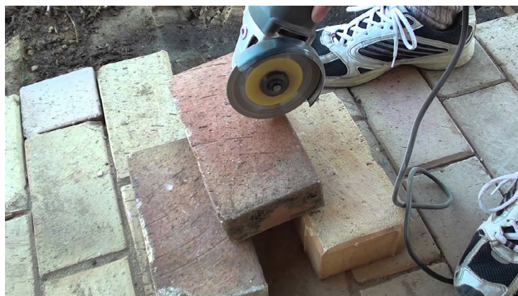
Fig. 5.1.15 Brick Cutting by Grinder
