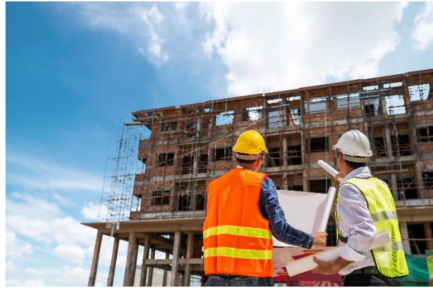
Fig. 1.1.5 Industrial Building Construction Site
