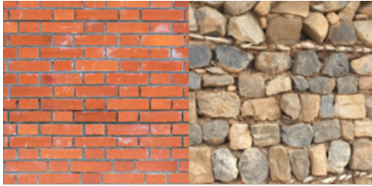
Fig.3.1.2 Brick and Stones Walls
