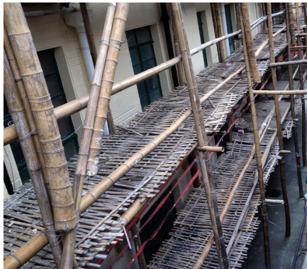
Fig. 2.2.5 Bamboo Scaffolding with working platforms
