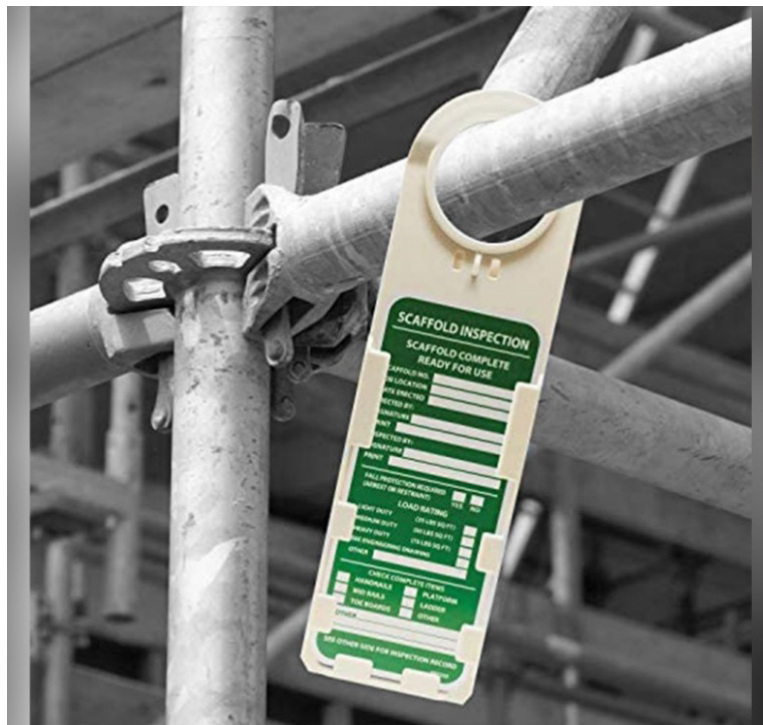
Fig.3.1.22 Inspected Scaffold
