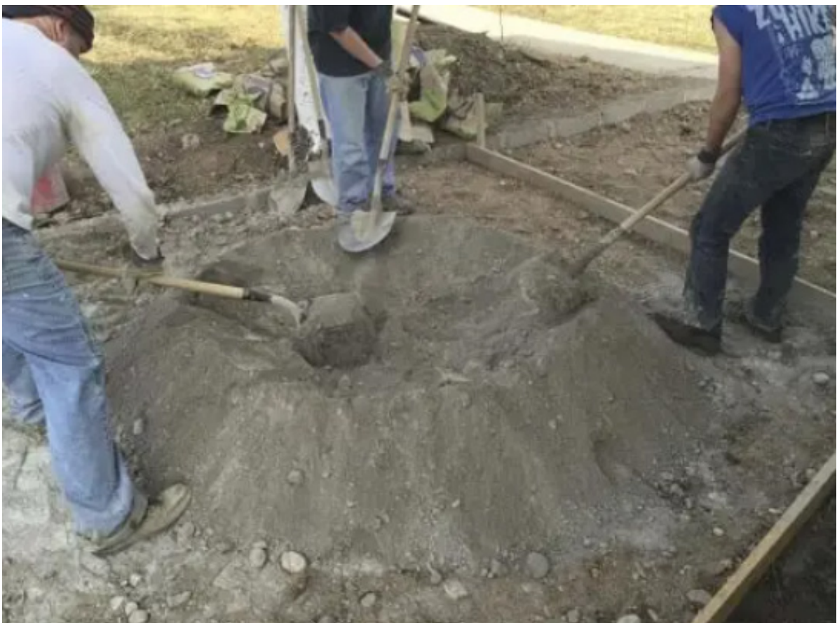
Fig. 4.3.2 Manual Mixing
