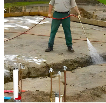
Fig. 1.2.4 Anti-Termite Solution
