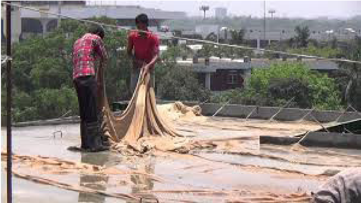
Fig. 4.2.11 Curing by Wet Fabrics
