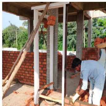
Fig. 1.2.9 Door and Window Fixing
