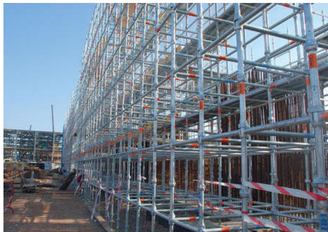
Fig. 2.3.1 Modular scaffolding system
