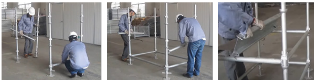
Fig. 2.4.2 Scaffolding work by mason
