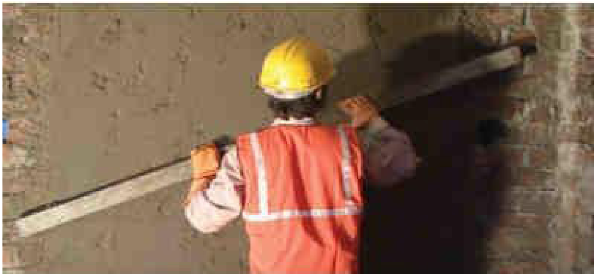
Fig. 5.2.1 Mason Plastering
