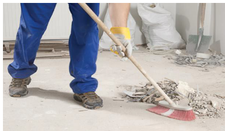
Fig. 7.3.5 Clean-up Debris and Waste
