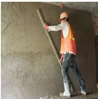
Fig. 1.2.8 Plastering
