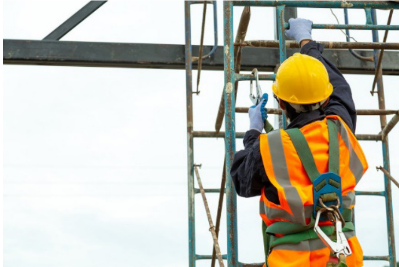
Fig.3.1.21 Construction Worker equipped with Fall Protection Equipment
