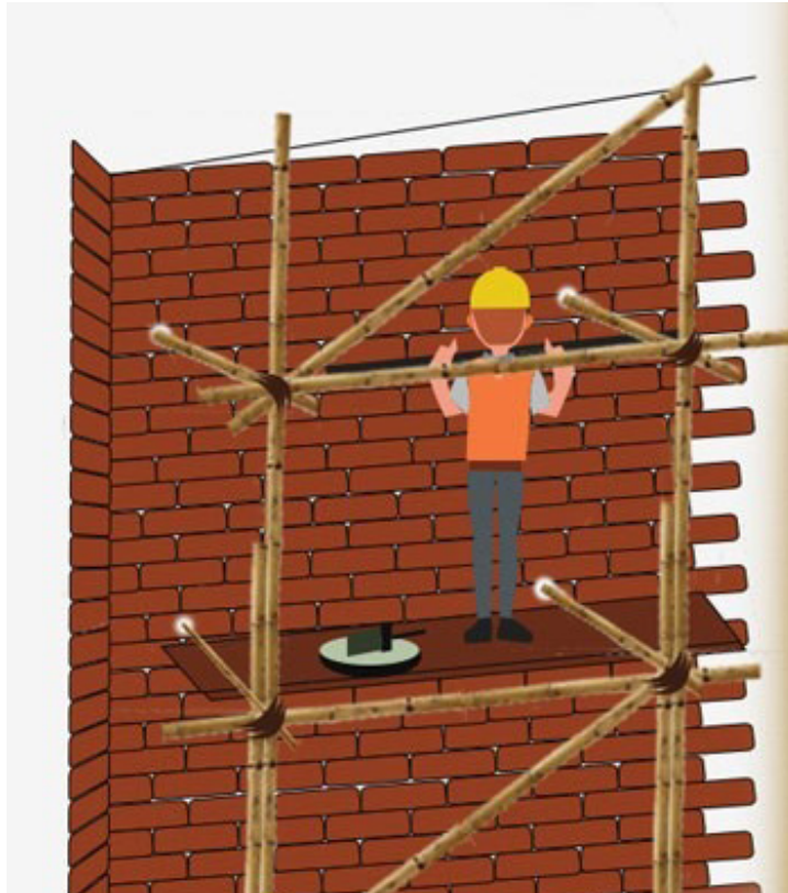
Fig. 2.2.8 Working on bamboo scaffolding
