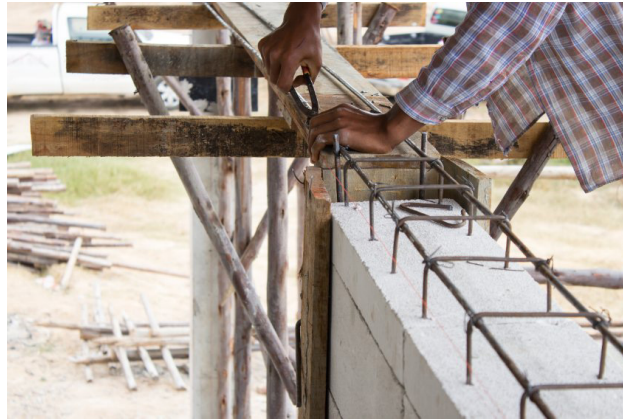
Fig.3.1.8 Reinforcement Work in Masonry
