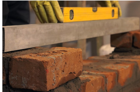
Fig.3.1.13 Process of using Spirit Level
