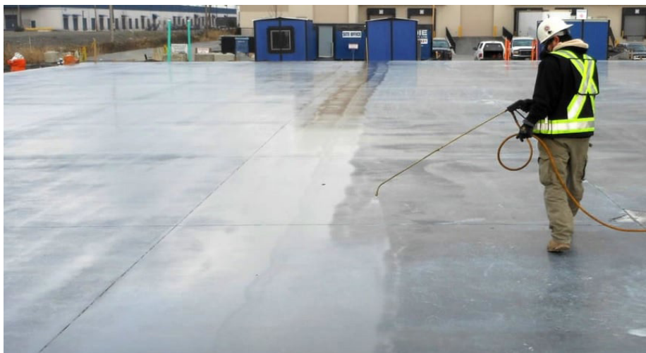
Fig. 4.2.11 Continuous Spraying
