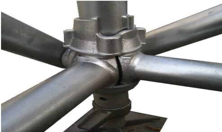
Fig. 2.3.3 Cuplock system scaffolding
