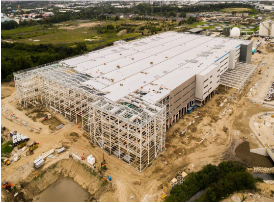
Fig. 1.1.4 Building Construction Site
