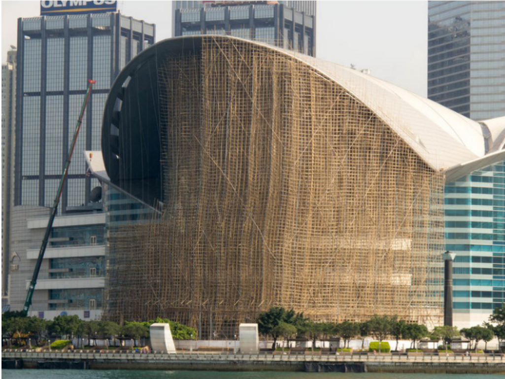
Fig. 2.2.6 Anchoring bamboo scaffold with building
