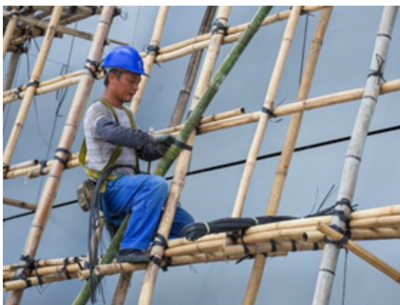
Fig. 2.2.1 Bamboo scaffolding
