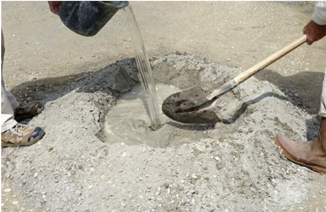
Fig.3.1.6 Mortar Preparation
