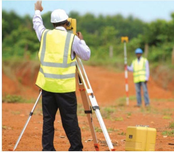
Fig. 3.2.1 Two-Person Method
