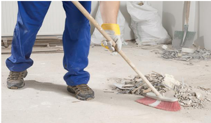
Fig. 5.3.5 Clean-up Debris and Waste
