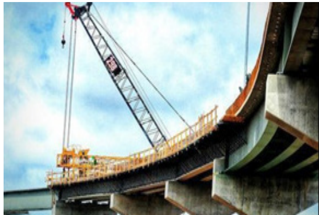
Fig. 1.1.2 under Construction Bridge
