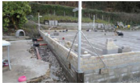
Fig. 3.3.3 Laying plumbing lines before survey
