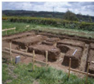
Fig. 3.3.2 Installing hurdles for marking
