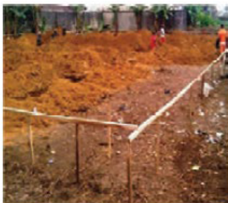
Fig. 3.3.1 Installing hurdles around excavation area
