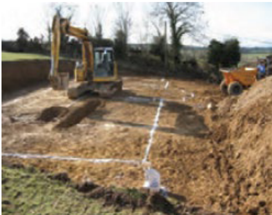
Fig. 3.3.9 Lime Application over Thread/Line Dory
