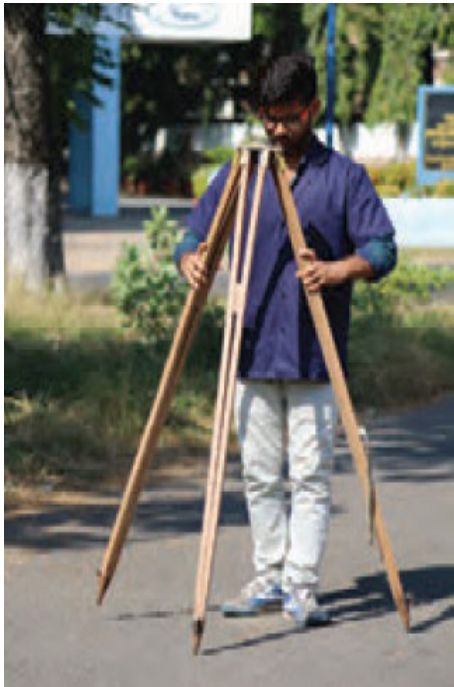
Fig. 3.1.5 Tripod fixed over the located point
