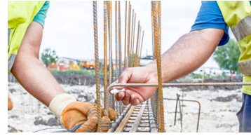
Fig. 4.1.1 Marking of rebar with a chalk
