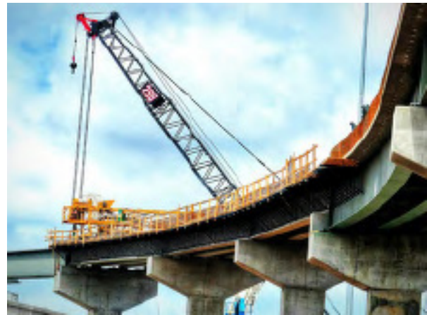
Fig. 1.1.2 Under Construction Bridge
