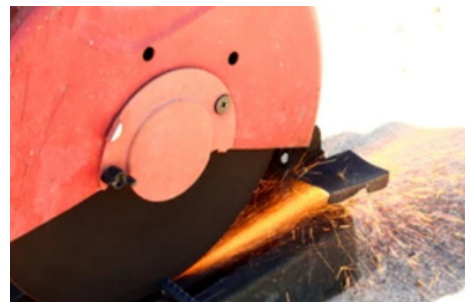
Fig. 3.1.1 Cutting of rebar
