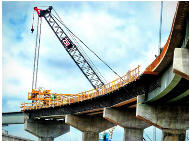
Fig. 1.1.2 Under Construction Bridge
