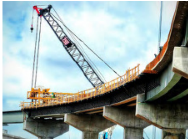
Fig. 1.1.2 Under Construction Bridge
