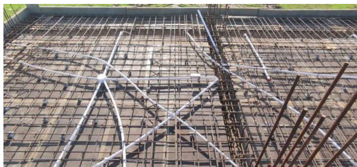
Fig. 4.1.13: Concealed Conduit in Slab
