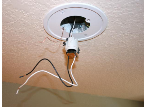
Fig. 4.1.17: Wiring and fitting fixture
