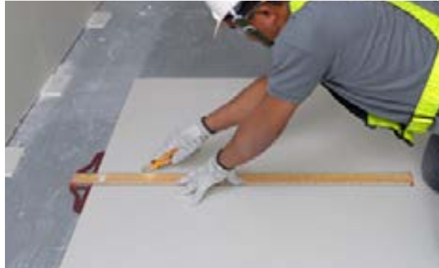
Fig. 4.1.11 Measuring and Cutting of the Board
