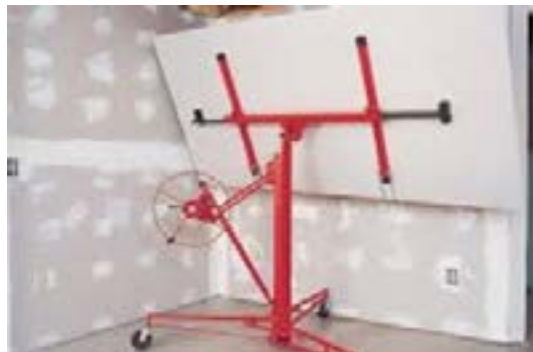
Fig. 4.1.14 Drywall Lifting using Hoisting
