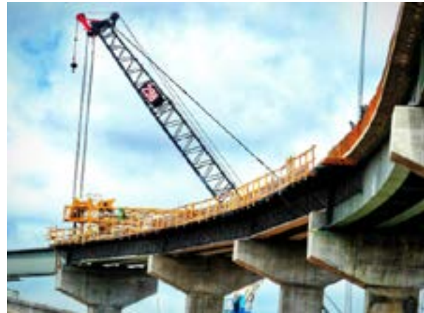
Fig. 1.1.2 Under Construction Bridge
