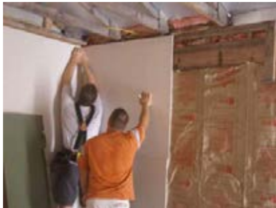
Fig. 4.1.13 Drywall Installation from Left top Corner
