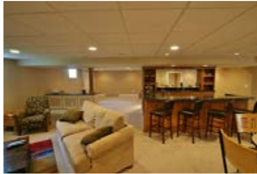
Fig. 4.1.6 Fiber False Ceiling
