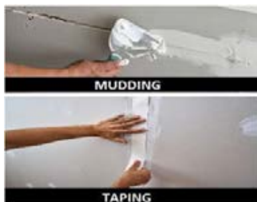
Fig. 4.1.15 Mudding and Taping
