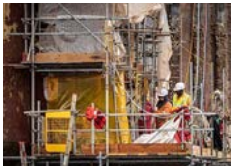
Fig. 1.1.4 Scaffolding at a construction site
