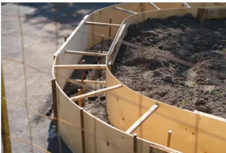
Fig. 2.1.3 Plywood Formwork
