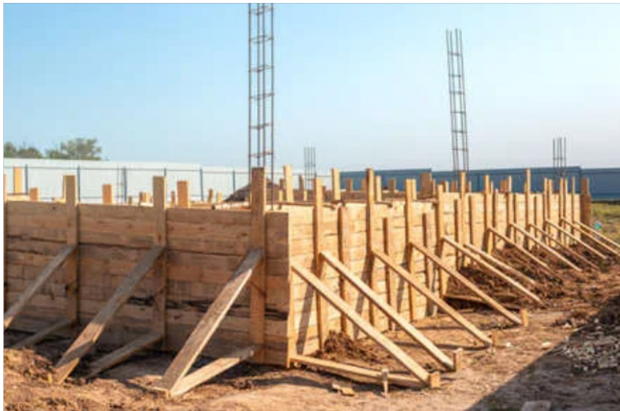
Fig 2.1.1 Timber Formwork
