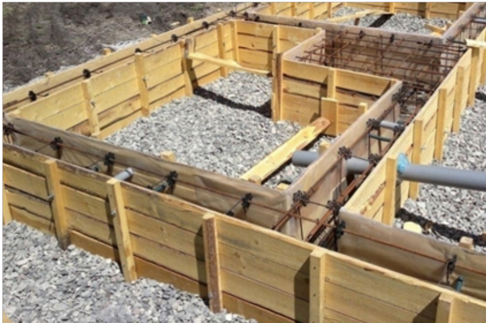
Fig. 3.1.1 Wooden Shuttering
