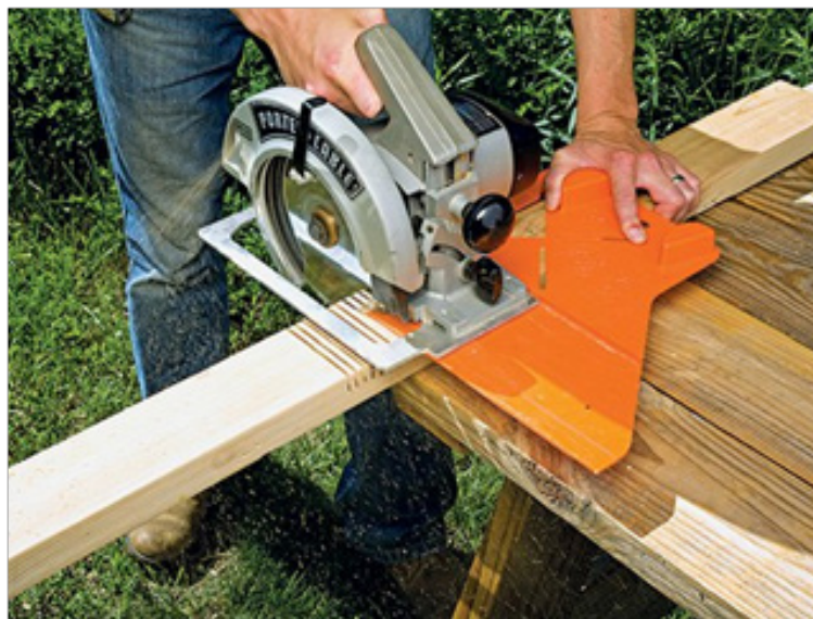
Fig. 3.1.13 Table Mounted Saw used for Cutting Shutter Boards
