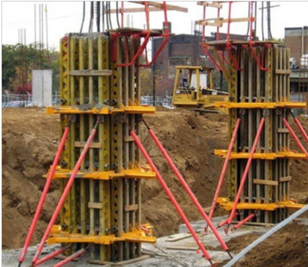
Fig 5.1.3 Formwork for Concrete Column Construction
