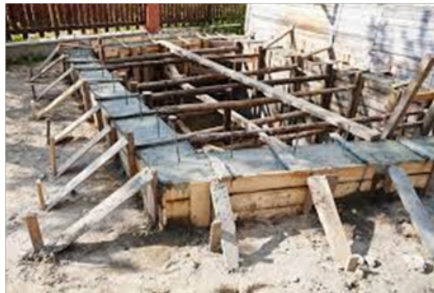
Fig. 3.1.3 Use of Wood Shuttering Board for Concrete
