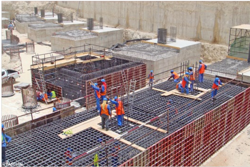
Fig. 5.1.1 On-going Work of Foundation Formwork
