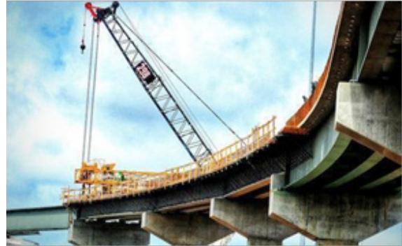
Fig. 1.1.2 Under Construction Bridge
