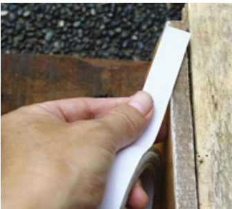
Fig 6.1.6 Masking of surface
