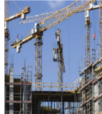
Fig 1.1.4 Industrial Building construction site
