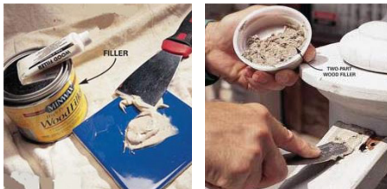
Fig 6.1.3 Applying wood filler on holes
