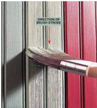
Fig 6.1.12 Applying second coat of paint
