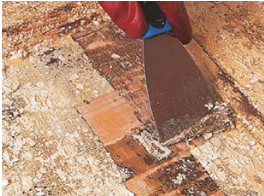
Fig 6.1.2 Removing old paint
