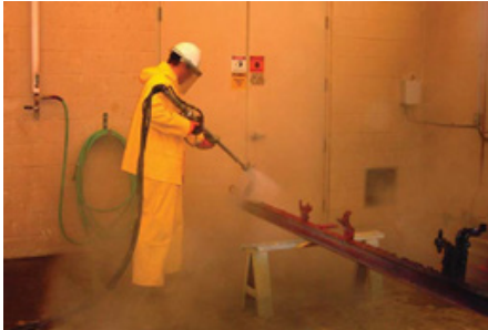
Fig 5.1.5 Jet washing of metal surface
