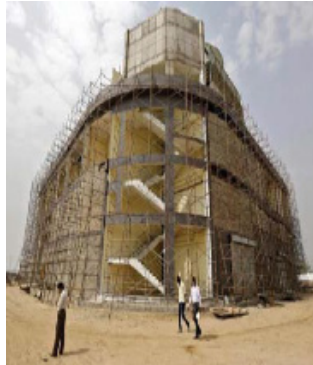
Fig 1.1.3 Building construction site
