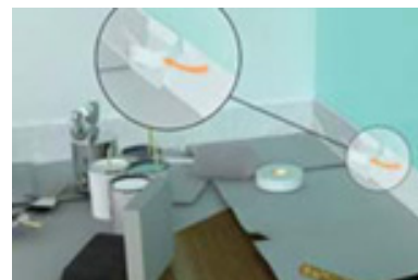
Fig 4.1.19 Removing masking tape
