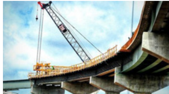
Fig. 1.1.8 Under Construction Bridge
