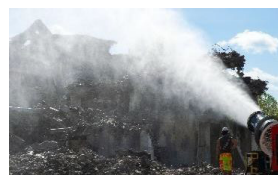
Fig. 10.3.10 Wetting Down Dust
