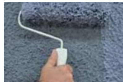
Fig 4.1.17 Applying paint using roller
