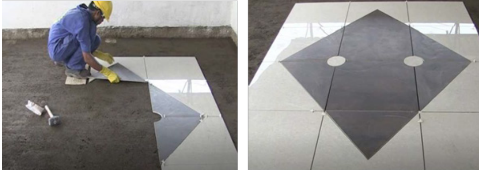
Fig. 9.1.6 Achieving Success in Tiling Work
