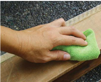
Fig 6.1.5 Cleaning surface by dry cloth
