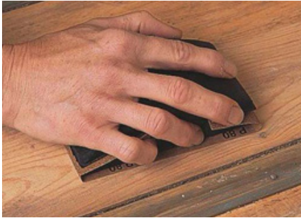
Fig 6.1.4 Sanding of surface
