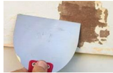
Fig 4.1.4 Scraping of surface
