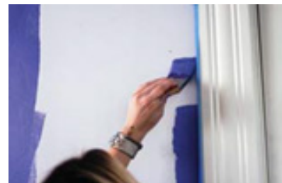
Fig 4.1.18 Applying paint using brush
