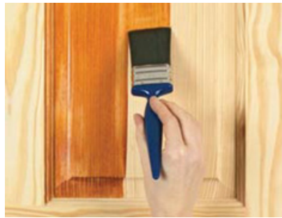
Fig 6.1.16 Applying varnish
