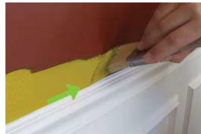
Fig 4.1.16 Applying paint on wall
