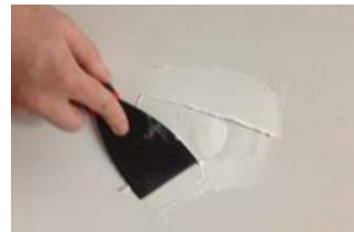
Fig 4.1.5 Applying putty on surface
