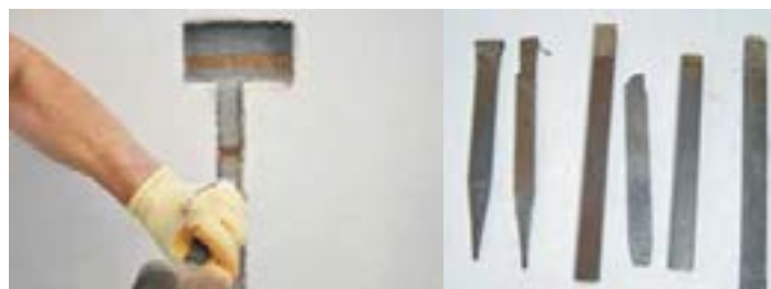
Fig. 3.1.18 Removing middle part
