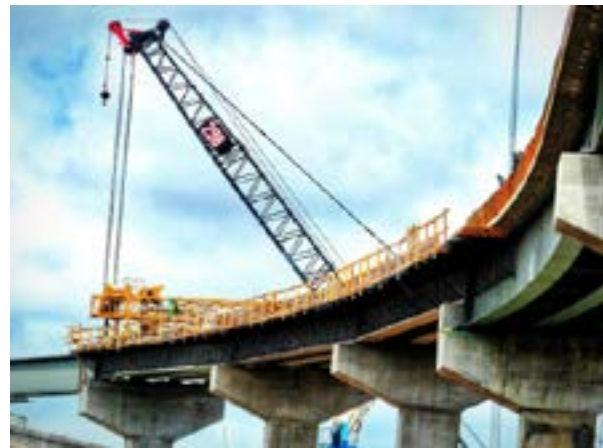
Fig. 1.1.2 Under Construction Bridge
