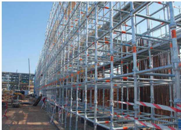
Fig. 5.3.1 Modular scaffolding system
