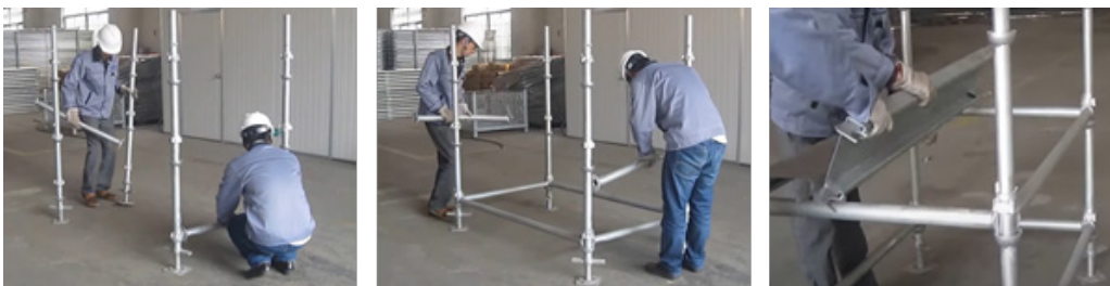
Fig. 5.4.2 Scaffolding work by mason
