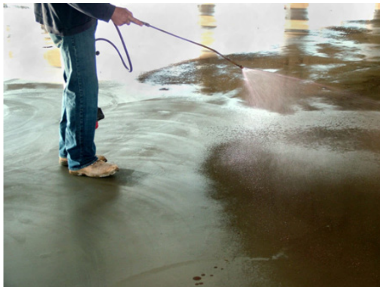
Fig. 6.2.6 Using curing agent/compound
