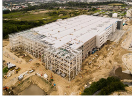
Fig. 1.2.5 Industrial Building Construction Site
