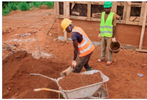
Fig. 4.1.7 Soil cutting
