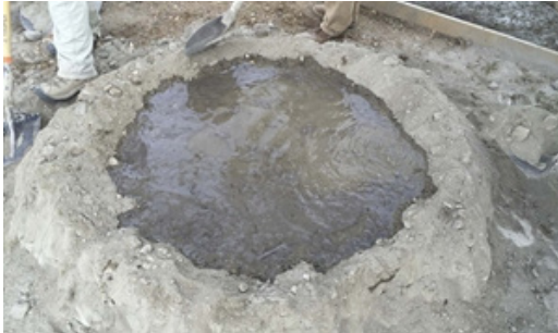
Fig. 6.1.3 Manual mixing
