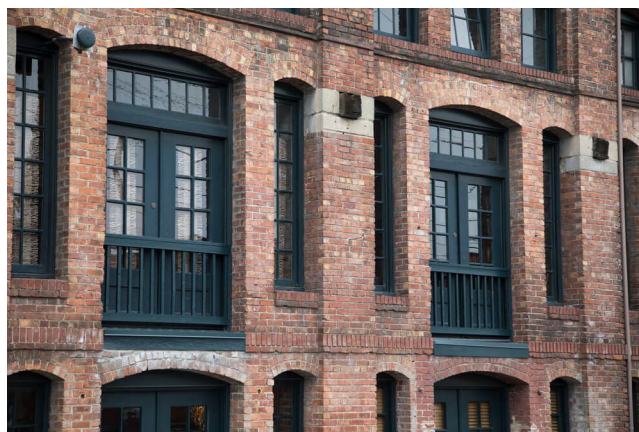
Bricks masonry used in building
