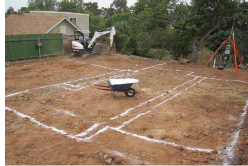
Step 2: Define the sides of the trench or pit using the point of spade.
