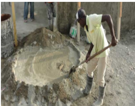
Fig. 1.3.7 Helper mason preparing cement mortar and curing by spraying water
