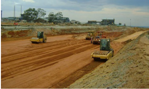
Fig. 4.1.3 Earth work for roads
