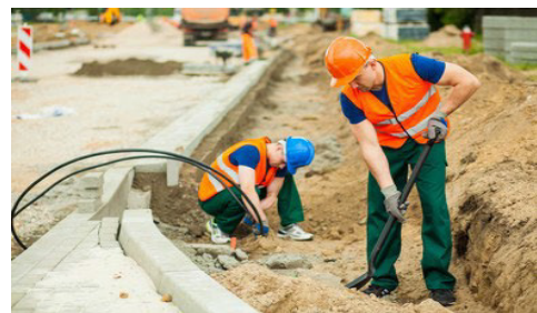
Step 6: Continue digging until the desired depth is not achieved.
