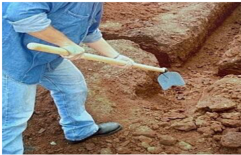
Step 3: Start digging using trenching hoe.
