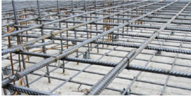
Fig. 1.2.12 Reinforcement bars fixed at site
