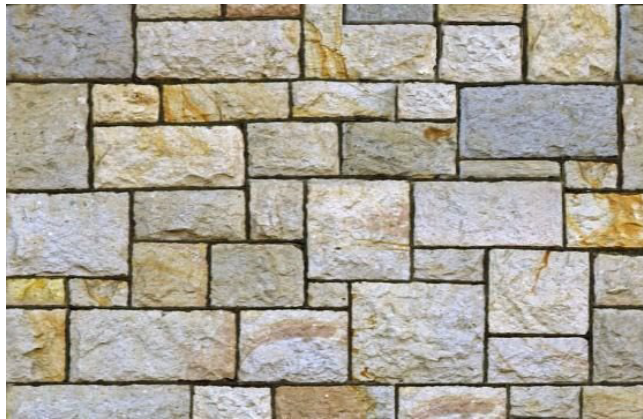
Rubble masonry in boundary wall
