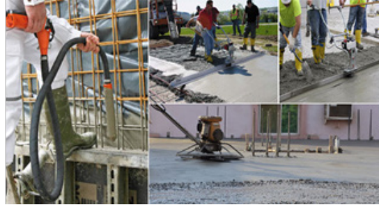
Fig. 4.2.4 Concrete compaction by vibrator
