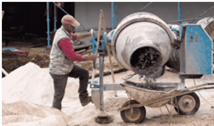
Fig. 6.1.8 Using hand-operated mixer
