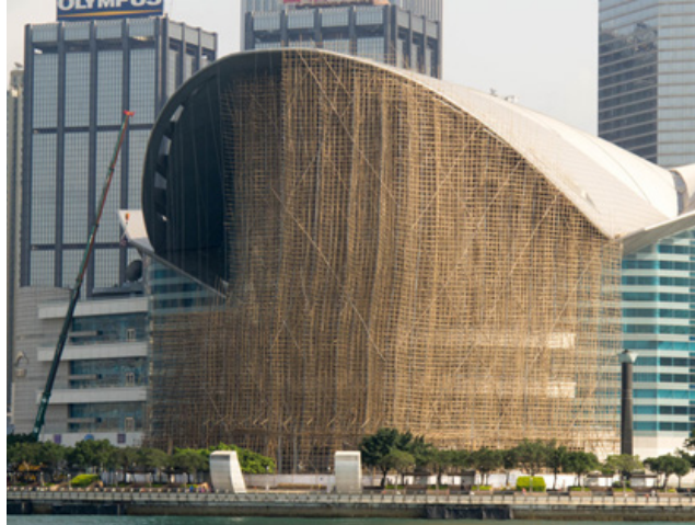
Fig. 5.2.6 Anchoring bamboo scaffold with building
