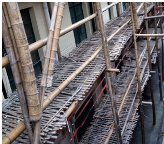
Fig. 5.2.5 Bamboo Scaffolding with working platforms
