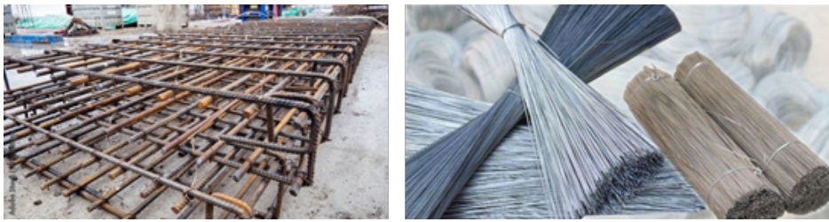
Fig. 3.2.27 Reinforcement bars and binding wires
