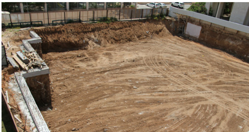
Fig. 4.1.11 Cutting soil manually
