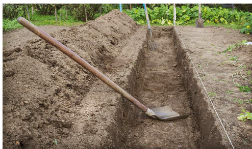
Step 5: Place all the soil that you pull out of the trench or pit on one side. This will leave the other side of the trench/pit easier to access. Dispose soil as per instructions.
