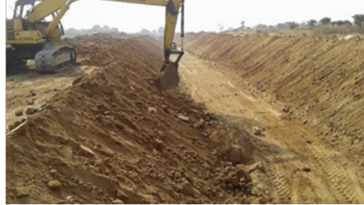
Fig. 4.1.4 Earth work for canals
