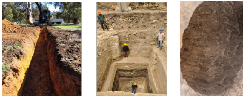
Fig. 4.1.9 Excavated trench and pit (large and circular)
