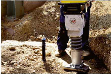
Fig. 4.2.3 Soil compaction by power rammer
