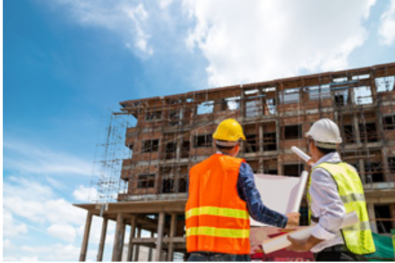
Fig. 1.2.4 Building Construction Site
