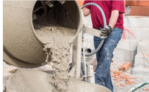
Fig. 6.1.4 Mechanical mixing
