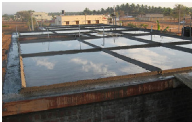
Fig. 6.2.3 Ponding method for curing of slab
