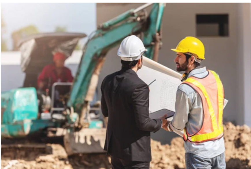
Fig. 4.1.10 Preparatory work prior to earthwork process
