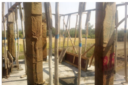
Fig. 6.2.5 Wet covering for curing
