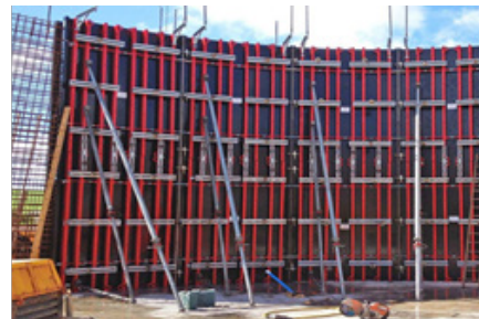
Fig. 1.2.14 System formwork
