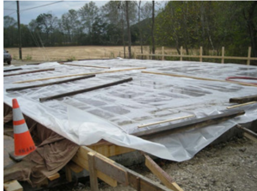
Fig. 6.2.4 Plastic sheets for curing of exposed concrete slab
