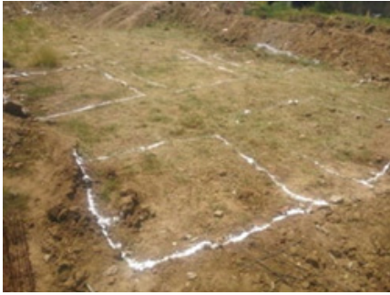
Fig. 4.1.6 Soil marking
