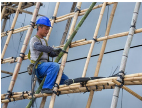
Fig. 5.2.1 Bamboo scaffolding
