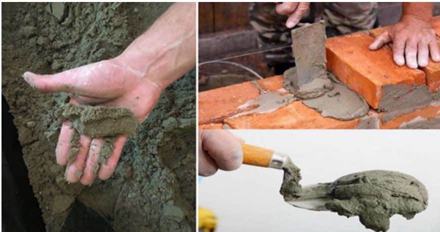
Fig. 3.2.18 Cement usage in masonry
