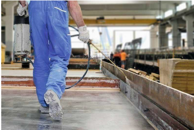
Fig. 3.4.11 Cleaning Mould and Applying the Oil/Mould release Agents
