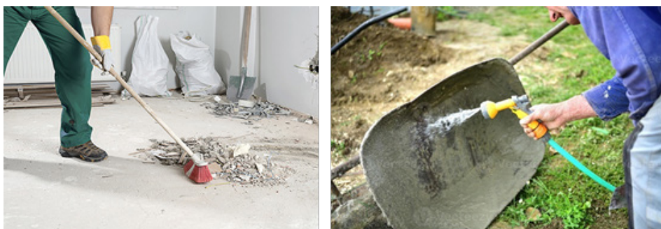
Fig. 1.3.10 Helper mason carrying out cleaning of debris/wastes and cleaning used tools
