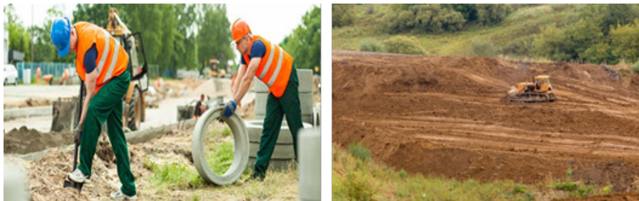
Fig. 4.1.5 Clearing the construction area
