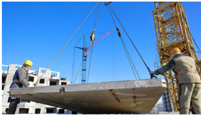
Fig. 1.2.17 Rigging work at site
