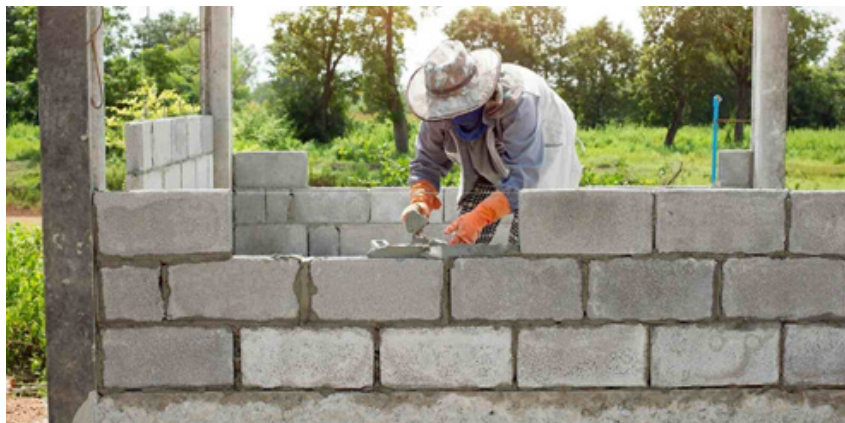
Fig. 1.3.3 Block masonry
