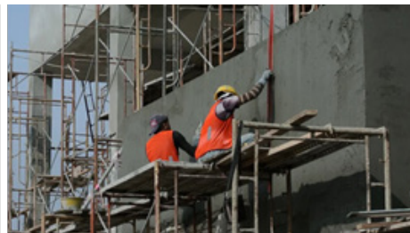
Fig. 1.2.10 Plastering Work
