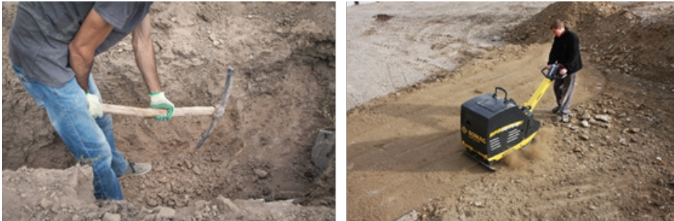
Fig. 1.3.8 Helper mason cutting/digging earth manually or performing compaction
