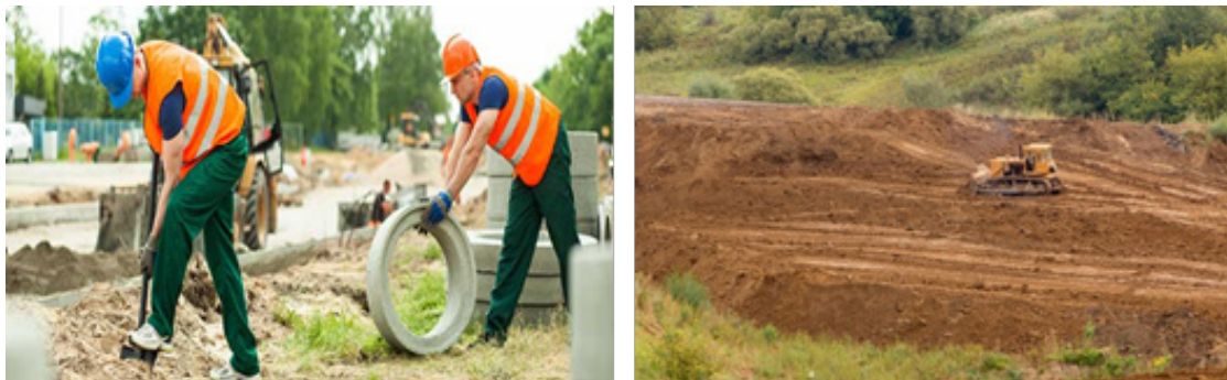
Fig. 4.1.5 Clearing the construction area
