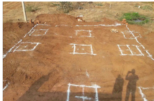
Step 6: Assist in the marking of layout.
