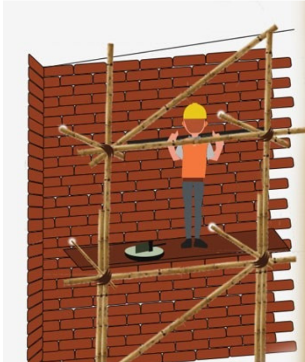
Fig. 5.2.8 Working on bamboo scaffolding
