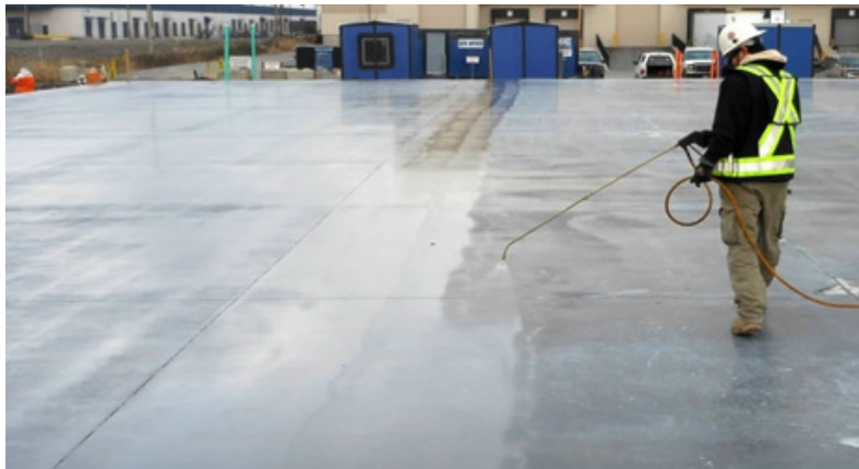
Fig. 6.2.2 Spraying of water for curing
