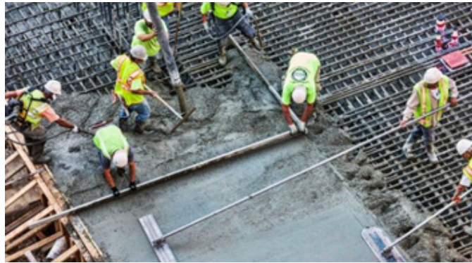
Fig. 3.3.1 Casting of RCC
