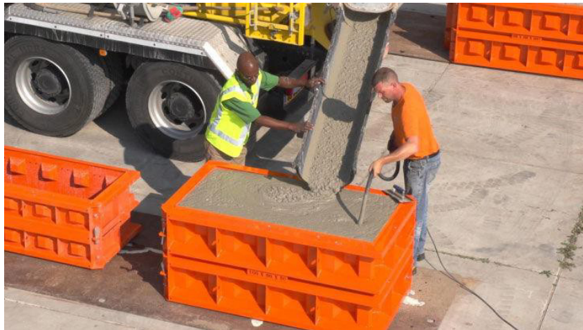
Fig. 3.4.15 Pouring Concrete in the Mould and Compacting
