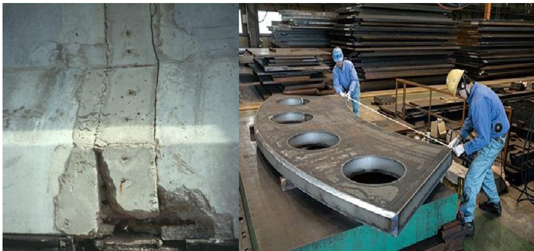
Fig. 3.4.17 Inspecting the precast structure for defects and measurement corrections
