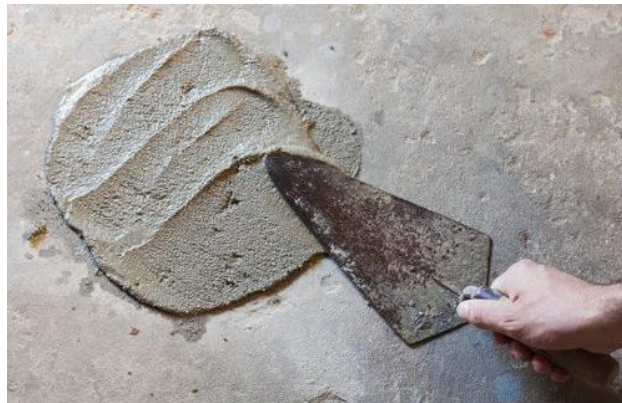
Fig. 3.5.4 Applying the mix over the area to be repaired
