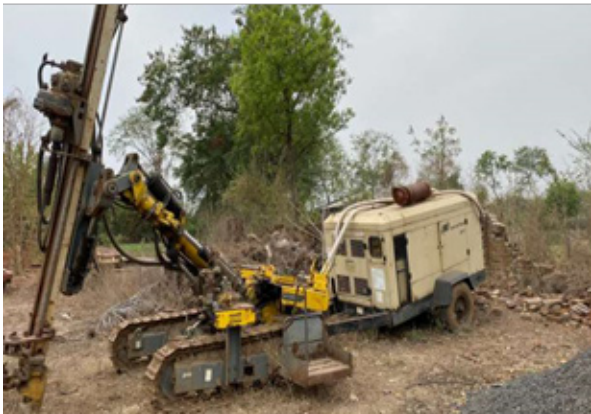
Fig. 1.2.7 Old Construction Equipment
