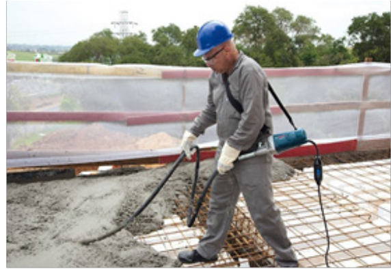
Fig. 1.3.8 Compacting Concrete using Vibrator
