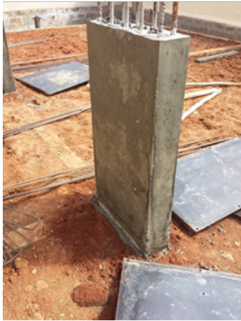
Fig. 3.3.25 De-shuttering
