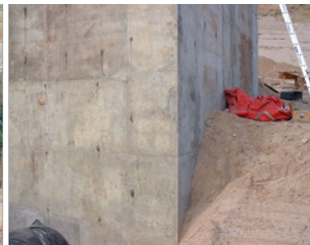
Fig. 3.3.34 Cured Concrete Wall
