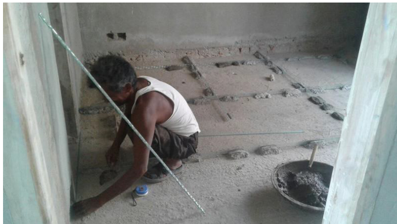
Fig. 4.2.1 IPS Flooring by Mason Concrete
