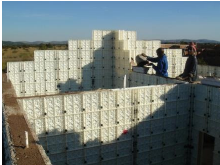
Fig. 3.3.6 Plastic Formwork
