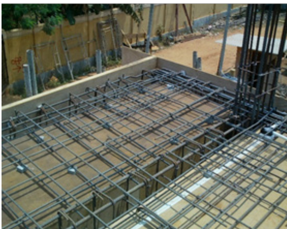
Fig. 1.2.11 Reinforcement bars fixed at site
