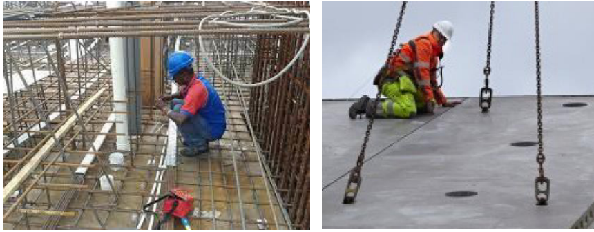
Fig. 3.4.13 Adding Pipe sleeves and lifting inserts
