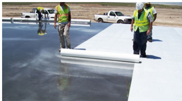
Fig. 3.1.25 Curing using plastic membrane
