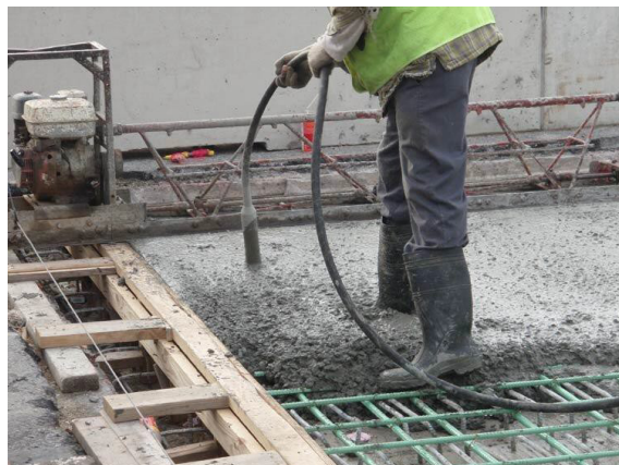
Fig. 4.1.11 Compacting using Needle Vibrator
