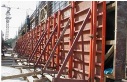
Fig. 3.3.4 Steel formwork
