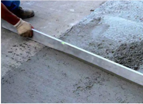
Fig. 3.1.20 Striking off concrete using straight edge
