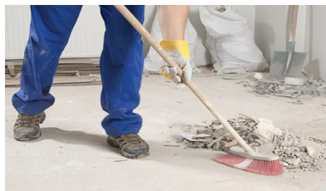
Fig. 7.3.5 Clean-up Debris and Waste
