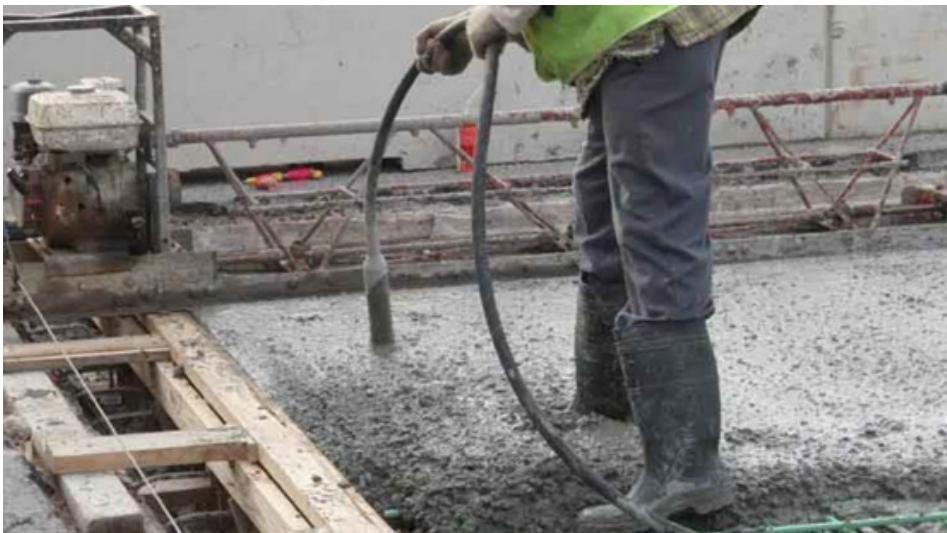
Fig. 3.2.4 Needle Vibrator
