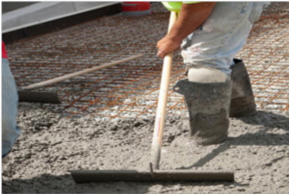
Fig. 1.3.7 Spreading Concrete
