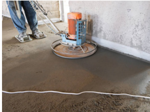
Fig. 3.2.9 Floating of newly formed Concrete Floor
