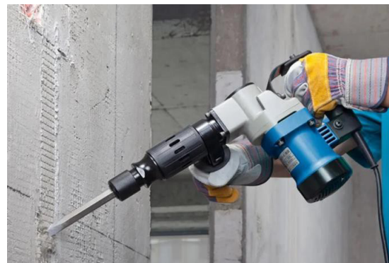
Fig. 3.5.3 Chipping Tools and Chipping using a Drill
