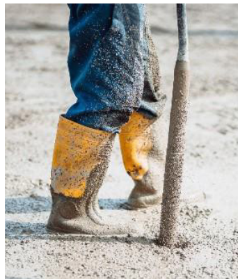
Fig. 3.3.45 Compacting
