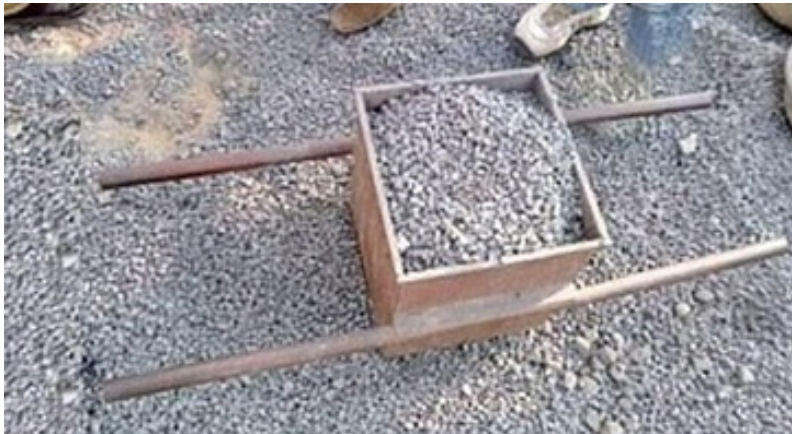
Fig. 3.1.9 Gauge Box used for Concrete Batching
