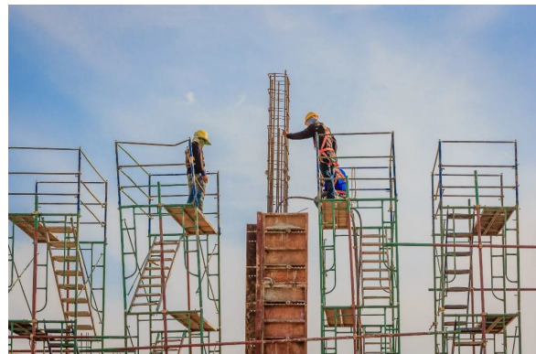
Fig. 5.1.4 Coordination during Construction Work
