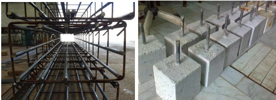
Fig. 3.4.12 Adding Rebars to the Mould
