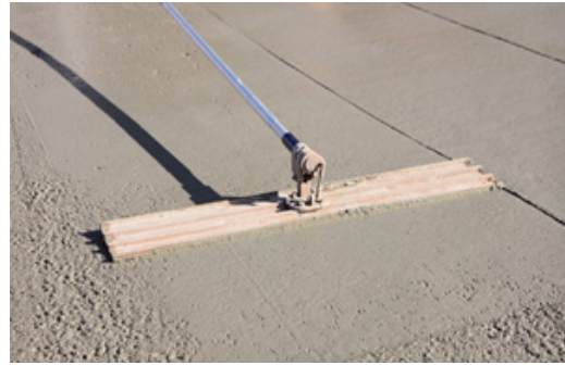
Fig. 3.1.21 Finishing concrete using bull float
