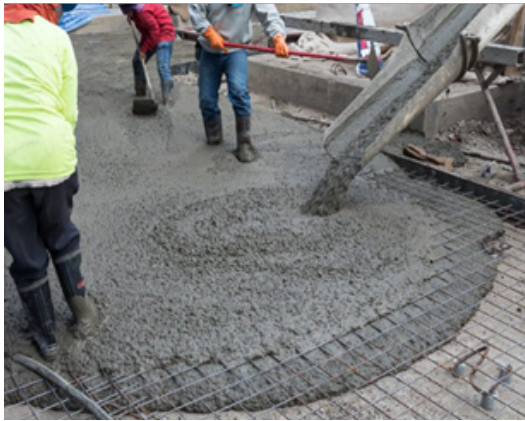
Fig. 1.2.9 Placing Concrete
