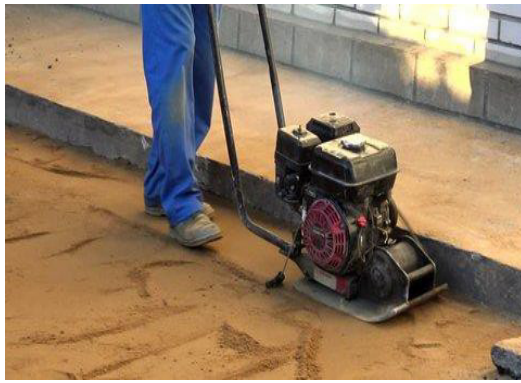
Fig. 4.1.3 Ramming of soil before subbase
