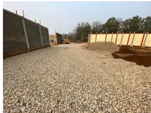
Fig. 4.1.5 Ramming of subbase
