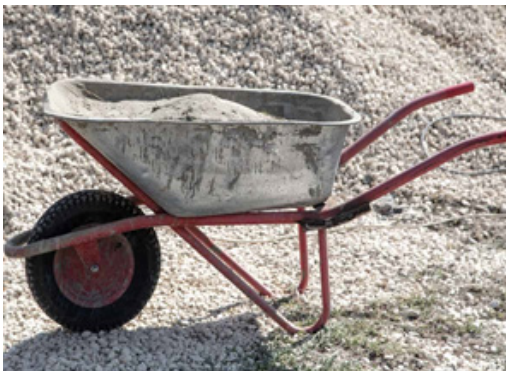
Fig. 3.1.15 Placing of Concrete by Wheelbarrow
