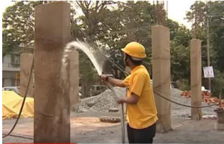
Fig. 3.1.24 Curing of concrete using water
