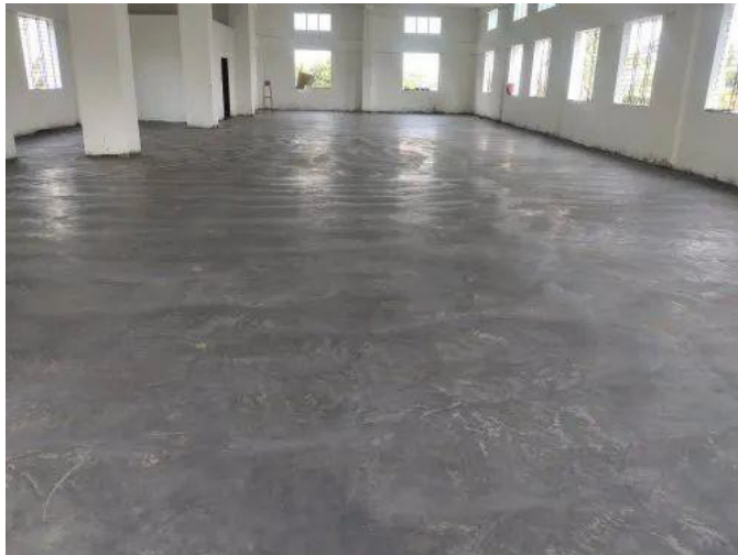
Fig. 4.3.4 Tremix Flooring Work
