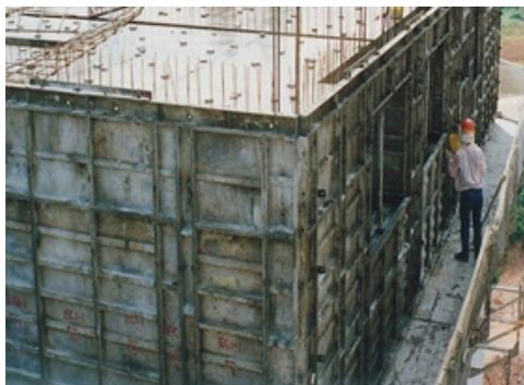
Fig. 3.3.33 De-shuttering
