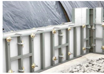
Fig. 3.3.5 Aluminium Formwork
