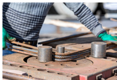
Fig. 3.3.13 Bending of Rebars
