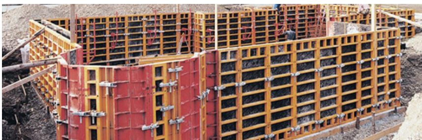
Fig. 3.3.2 Plywood Formwork
