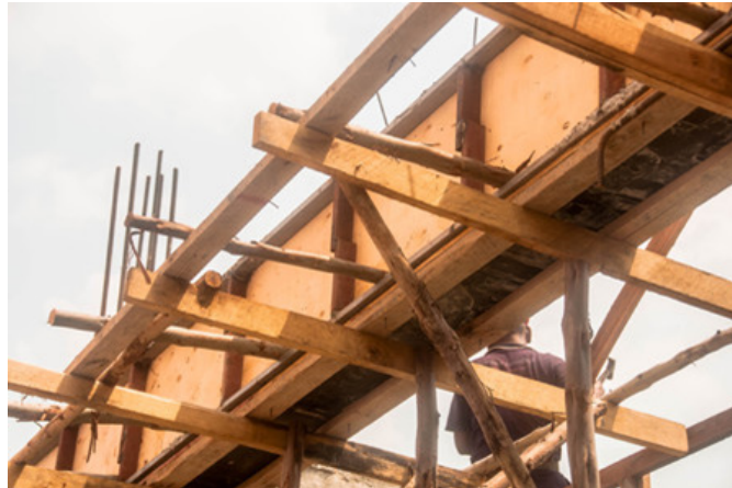
Fig. 3.3.3 Timber form work
