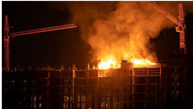
Fig. 7.2.3 Fire at Construction Site
