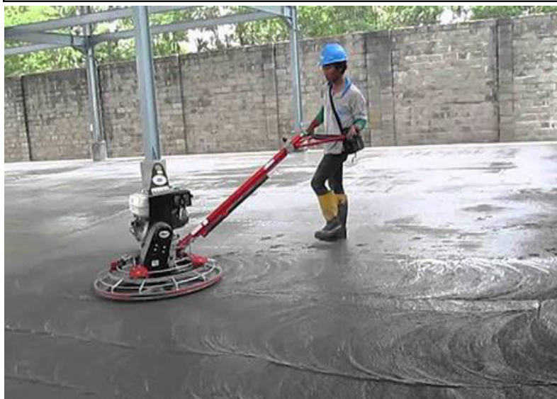
Fig. 4.3.5 Vacuum de-watering for Tremix Flooring
