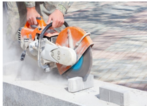
Fig. 3.2.11 Cutting concrete using Concrete Saw
