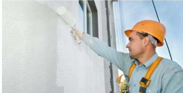
Fig. 1.2.16 Paint work by a painter
