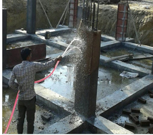
Fig. 3.3.26 Cured concrete Column
