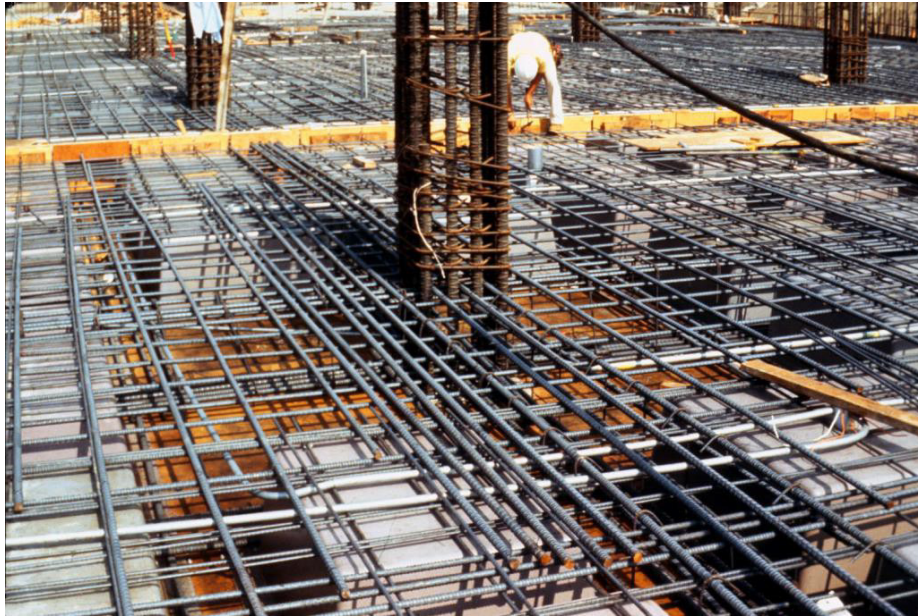
Fig. 4.1.10 Rebar used for reinforcement
