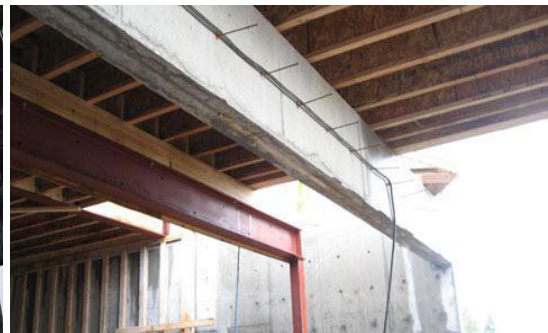
Fig. 3.3.48 Cured Concrete Beam
