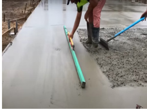
Fig. 3.2.6 Screeding of Newly Formed Concrete Floor
