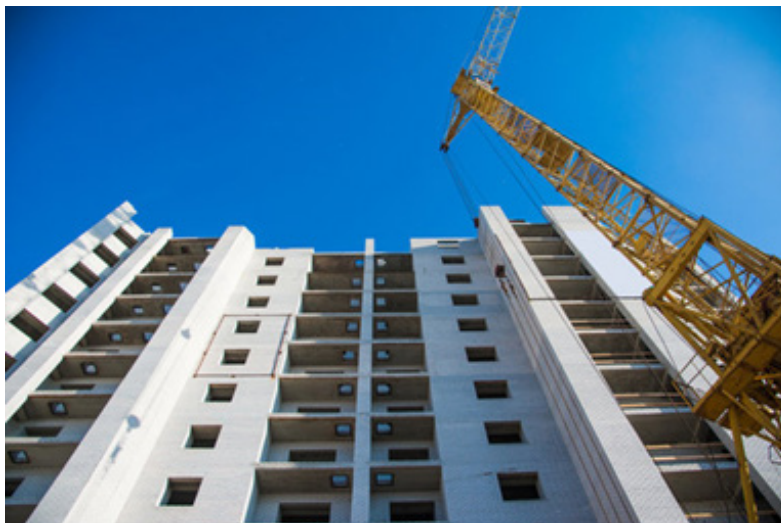
Fig. 1.2.1 Multi Storey Residential Towers
