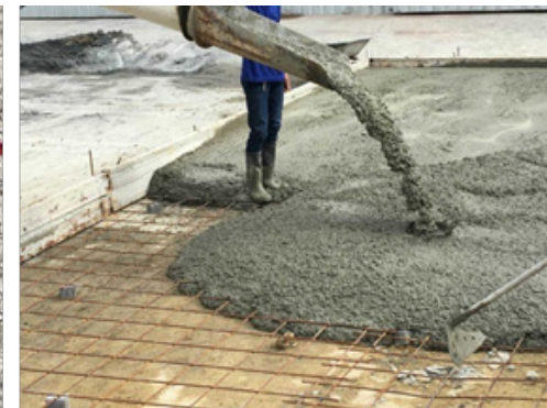
Fig. 3.1.16 Placing of Concrete by Chute
