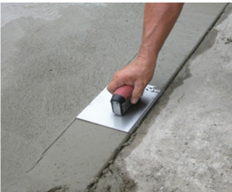
Fig. 3.1.22 Finishing concrete using edging trowel
