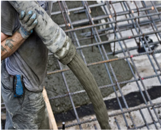
Fig. 3.1.17 Pouring of Concrete by Pump
