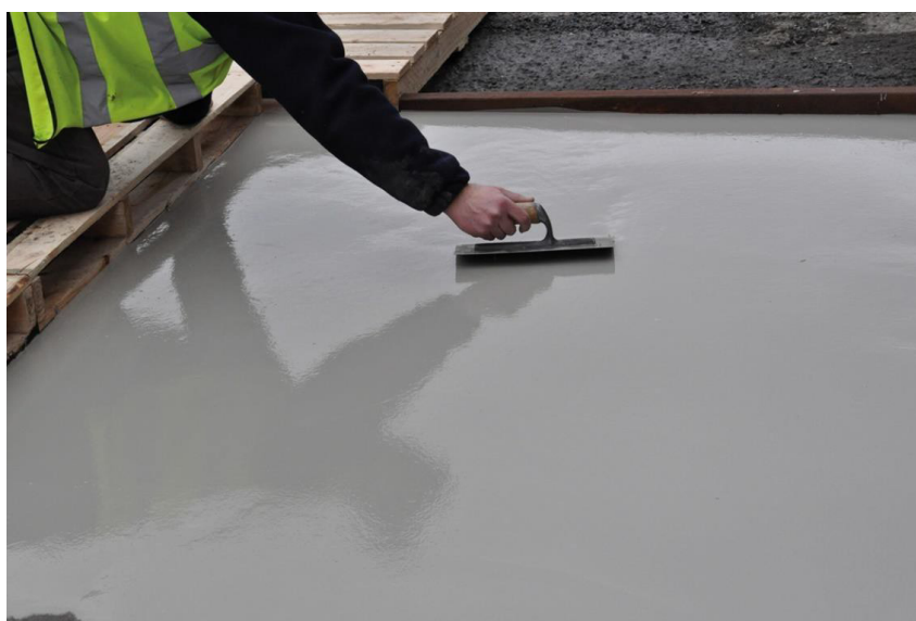
Fig. 3.4.16 Screeding of Poured Concrete
