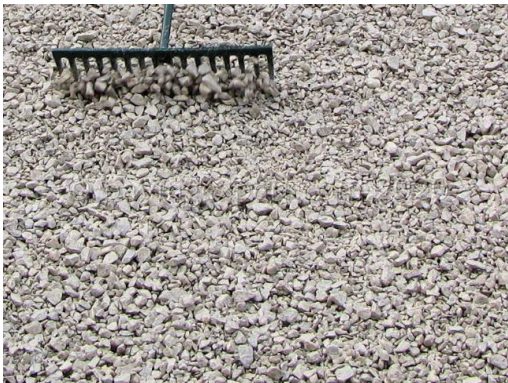
Fig. 4.1.4 Open grade stone used as subbase
