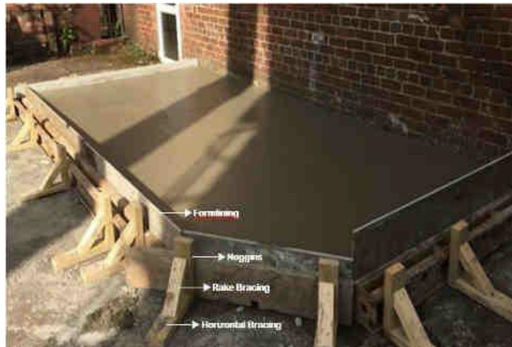
Fig. 4.1.8 Concrete flooring using Timber Shuttering
