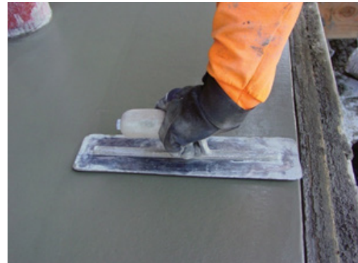
Fig. 3.1.23 Finishing concrete using concrete trowel
