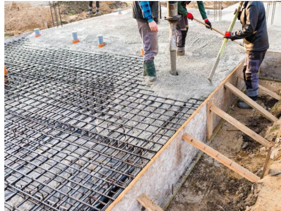
Fig. 3.3.38 Compacting
