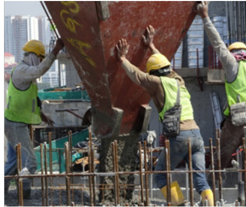
Fig. 3.1.18 Pouring of Concrete by Tower Crane
