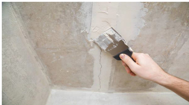
Fig. 3.5.5 Repairing Defects in the Ceiling Area
