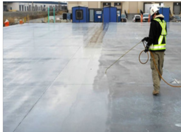
Fig. 1.3.10 Curing Concrete by Water Spray
