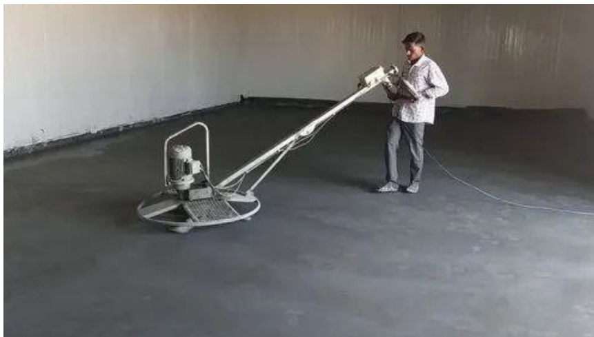
Fig. 4.3.7 Power trowel for trowelling of hardened concrete for smooth finish
