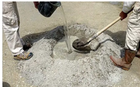
Fig. 3.1.12 Manual Concrete Mixing
