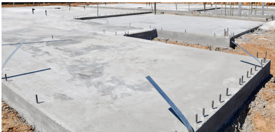
Fig. 3.3.41 Concrete Foundation after De-shuttering
