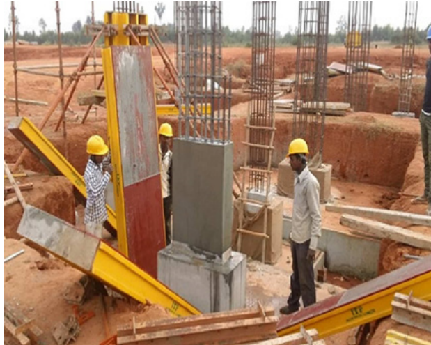
Fig. 3.3.19 Removal of Formwork
