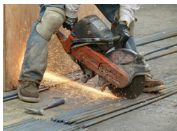
Fig. 3.3.12 Cutting of Rebars
