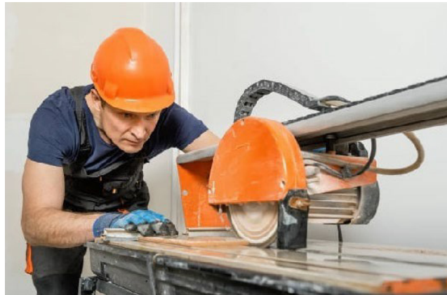
Fig. 4.2.11: Positioning tile on the wet saw
