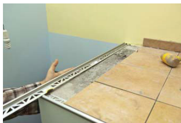
Fig. 4.3.31: Screwing and placing trim edges
