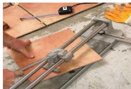
Fig. 4.2.10: Cutting tile by the machine
