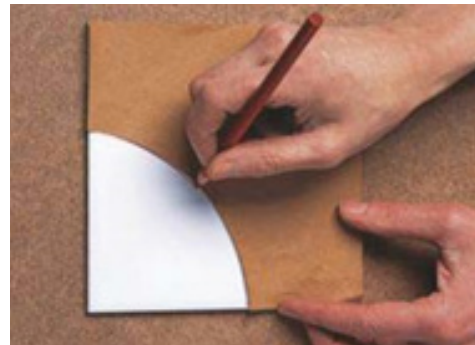
Fig. 4.2.6: Marking curves on tile
