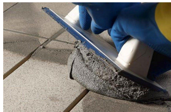
Fig. 5.1.4 Applying grout on joints
