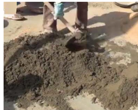
Fig. 4.3.20: Preparing mortar
