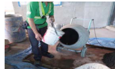
Fig. 4.3.14: Adding water in mixer
