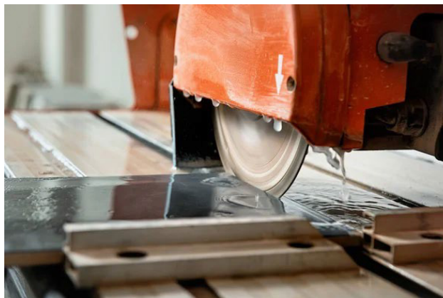
Fig. 4.2.12: Cutting tile by wet saw
