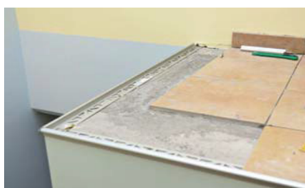
Fig. 4.3.32: Installing trim edges
