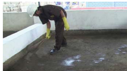
Fig. 4.3.1: Cleaning surface by broom
