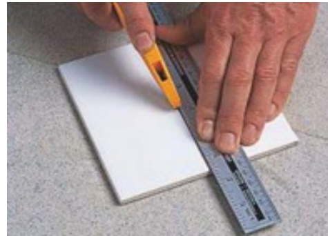
Fig. 4.2.4: Marking on tile by steel rule
