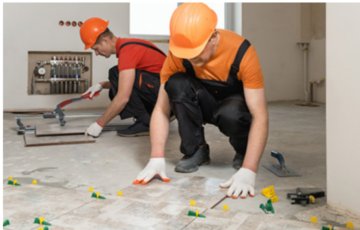
Fig. 1.3.1 Mason Tiling performing the work
