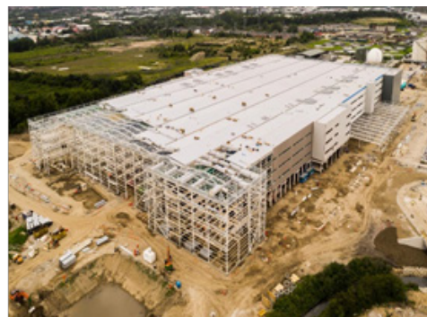
Fig. 1.1.5 Industrial Building Construction Site
