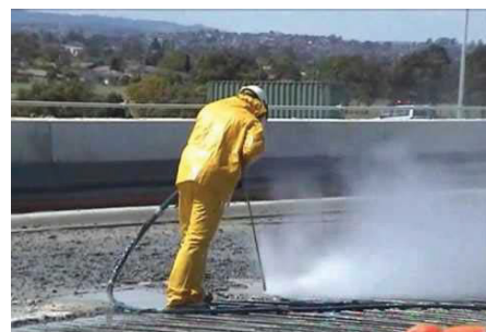
Fig. 4.3.2: High pressure water blasting
