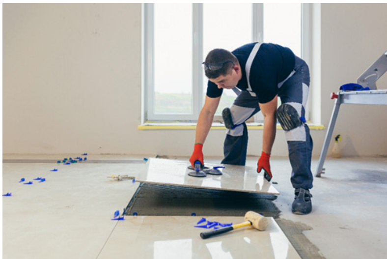
Fig. 1.3.3 Placing tiles on the surface
