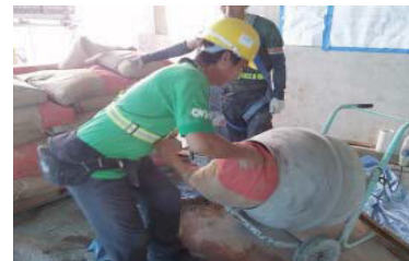
Fig. 4.3.13: Adding cement in mixer
