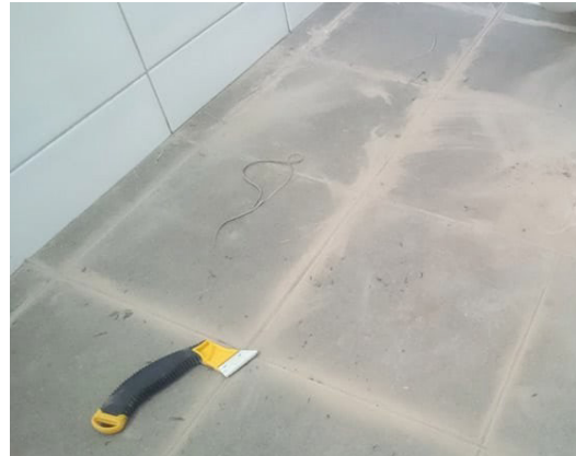
Fig. 5.1.7 Grout removal tool
