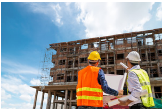
Fig. 1.1.4 Building Construction Site
