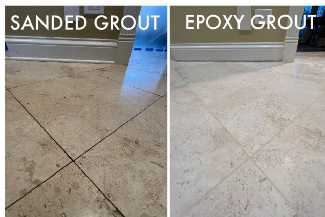
Fig. 3.2.10: Sanded and epoxy grout
