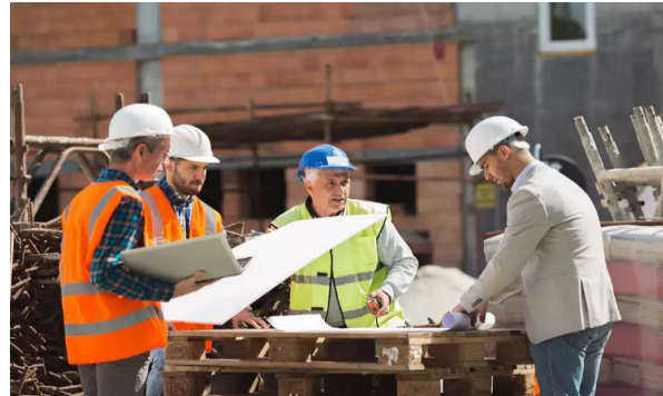
Fig. 6.1.3 Communication at Construction
