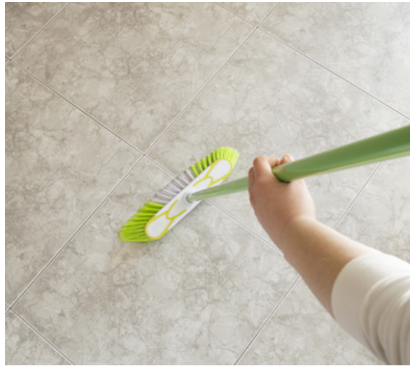
Fig. 5.2.3 Mopping after curing of grout
