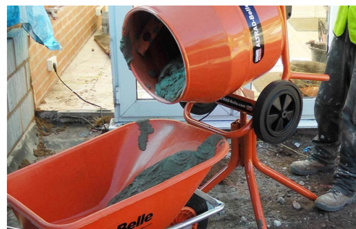
Fig. 4.3.11: Prior wet mixing wheelbarrow and mixer
