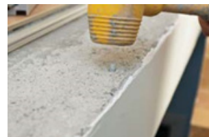
Fig. 4.3.30: Inserting dowels in surface
