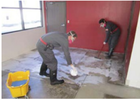
Fig. 4.3.3: Acid etching
