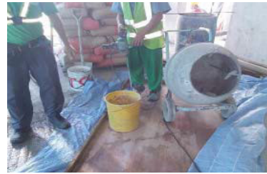
Fig. 4.3.12: Preparing mixture and bucket
