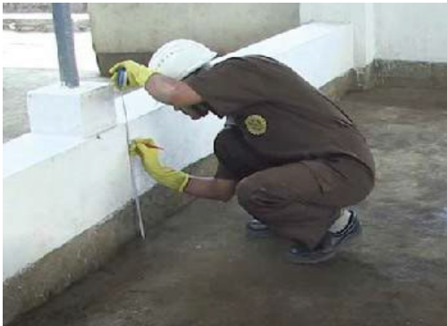
Fig. 4.3.21: Measuring and marking on wall
