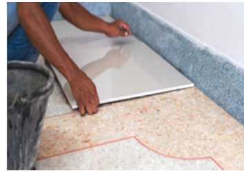
Fig. 4.3.24: Placing first tile for reference
