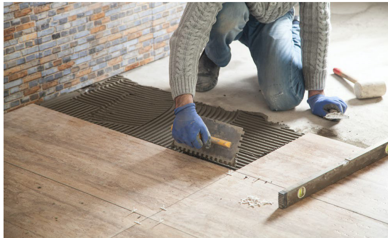
Fig. 3.2.11: Proper tile installation
