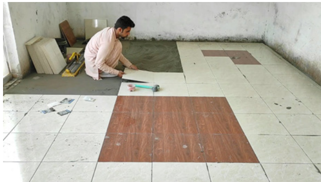
Fig. 7.3.1 Mason Tiling doing tiling Work
