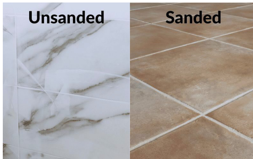
Fig. 3.2.9: Unsanded and sanded Grout
