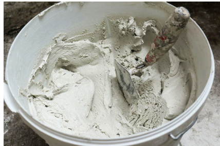
Fig. 5.1.1 Mixing grout by trowel
