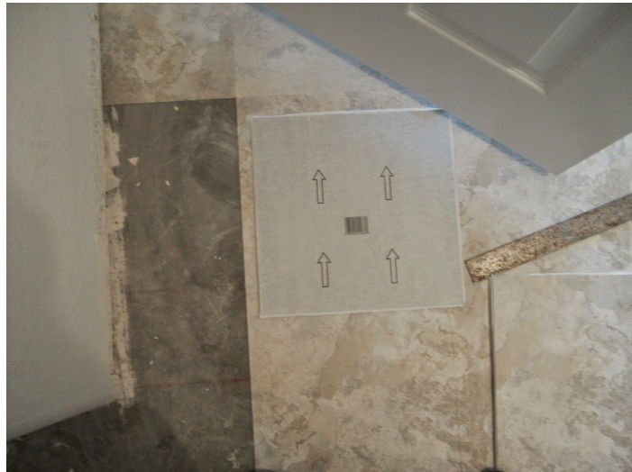
Fig. 4.2.3: Direction marks for the tile
