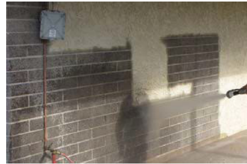
Fig. 4.3.4: Sand blasting
