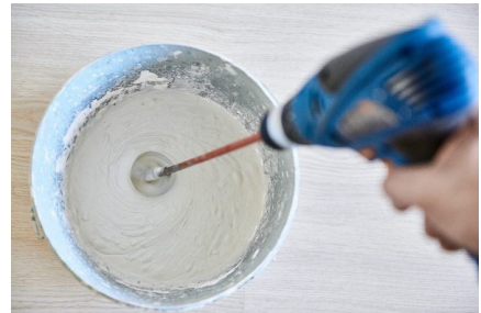
Fig. 5.1.2 Mixing grout by handheld mixer
