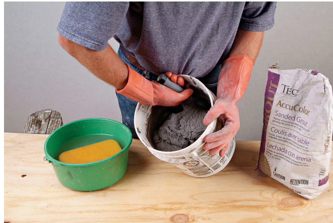
Fig. 5.1.3 Checking of grout
