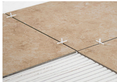
Fig. 4.3.25: Placing tile spacers
