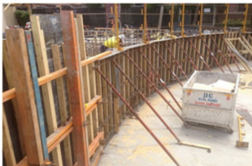
Fig. 1.2.5 Conventional formwork
