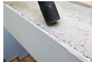
Fig. 4.3.29: Cleaning surface
