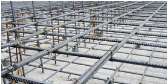
Fig. 1.2.3 Reinforcement bars fixed at site
