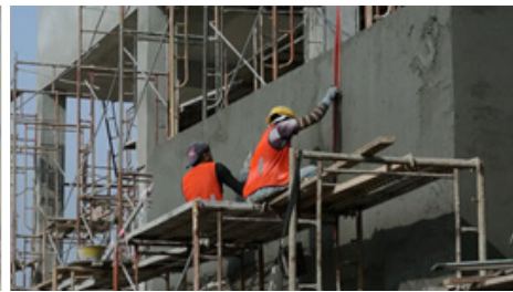
Fig. 1.2.2 Plastering Work
