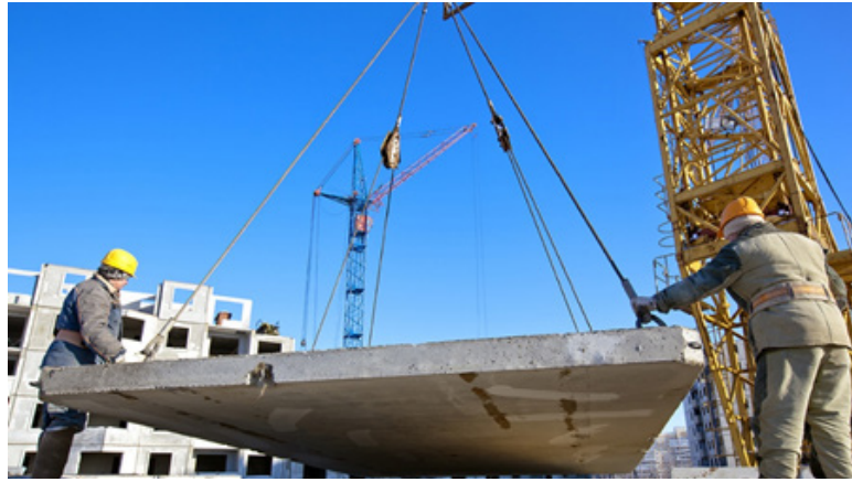
Fig. 1.2.9 Rigging work at site
