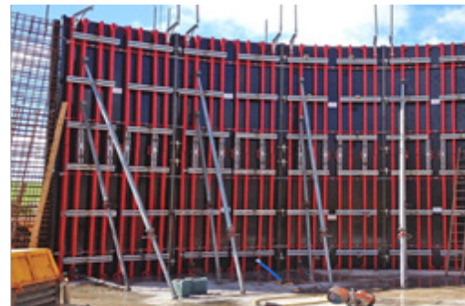
Fig. 1.2.6 System formwork
