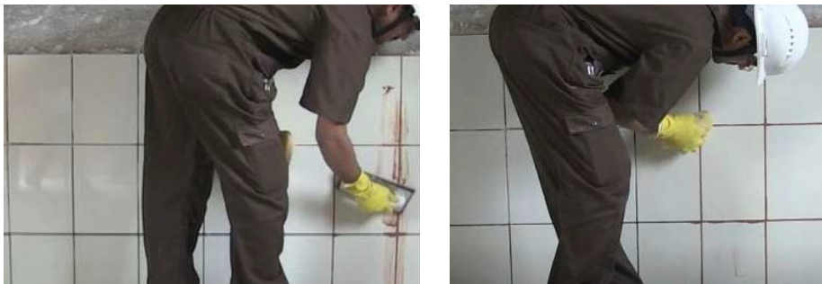
Fig. 5.1.5 Mason tiling at work
