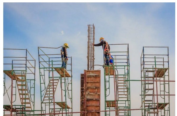
Fig. 6.1.4 Coordination during Construction Work
