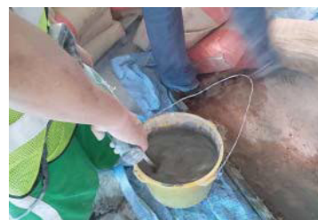
Fig. 4.3.16: Mixing of mortar by hand mixer
