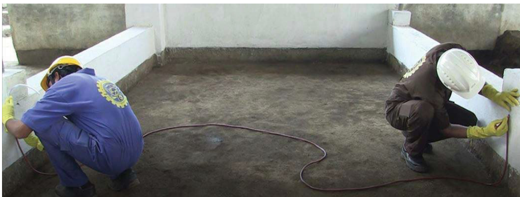
Fig. 4.3.22: Marking prior to tile layout
