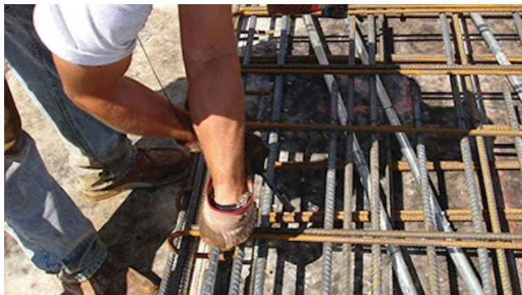
Fig. 4.1.5 Maintain integrity of reinforcement bars during the straightening process
