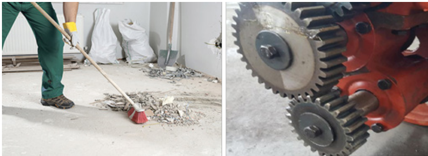
Fig. 1.2.8 Carrying out cleaning of debris/wastes and cleaning used tools
