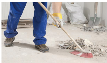
Fig. 7.3.5 Clean-up Debris and Waste
