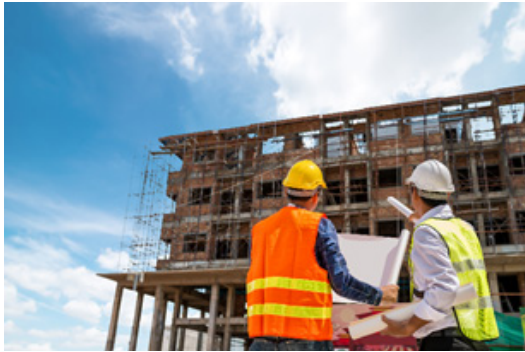
Fig. 1.1.4 Building Construction Site
