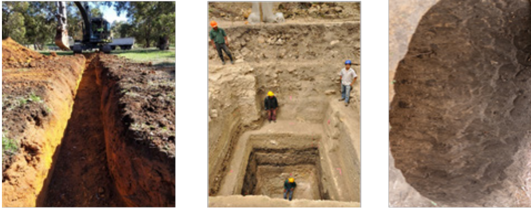
Fig. 9.1.9 Excavated trench and pit (large and circular)
