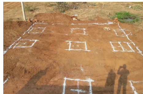
Step 6: Assist in the marking of layout.
