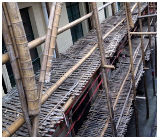
Fig. 6.2.5 Bamboo Scaffolding with working platforms
