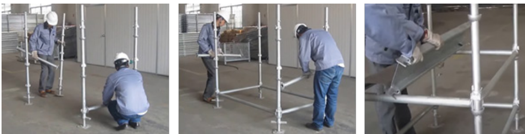
Fig. 6.4.2 Scaffolding work by mason
