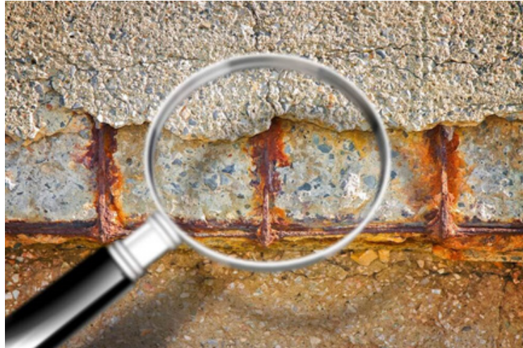
Fig. 3.1.40 Prevent reinforcement corrosion
