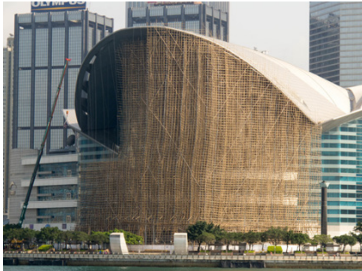
Fig. 6.2.6 Anchoring bamboo scaffold with building
