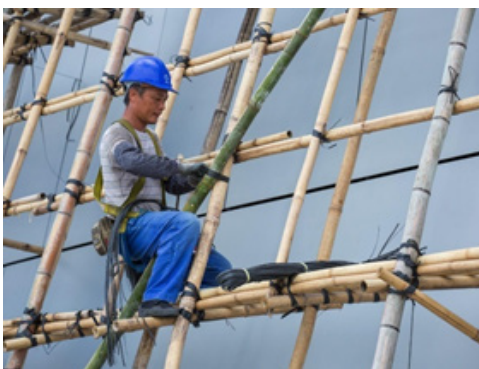
Fig. 6.2.1 Bamboo scaffolding
