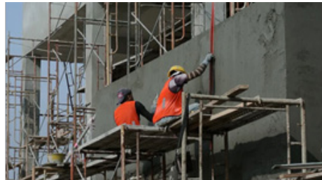
Fig. 1.1.10 Plastering Work
