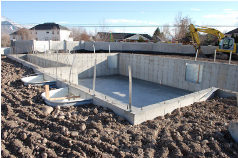
Fig. 9.2.2 Backfilling
