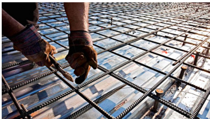
Fig. 5.1.1 Proper tying of reinforcement bars
