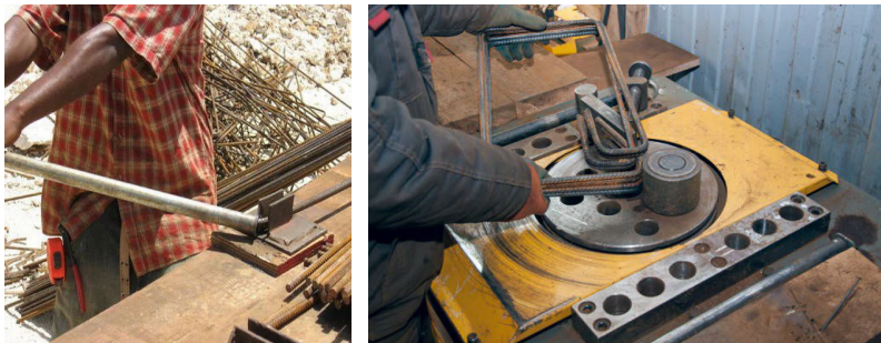
Fig. 1.2.4 Bending of a rebar
