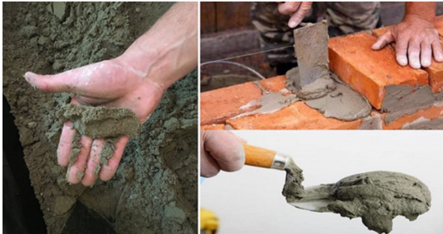
Fig. 3.1.18 Cement usage in masonry
