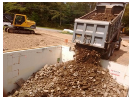
Fig. 9.1.2 Back filling
