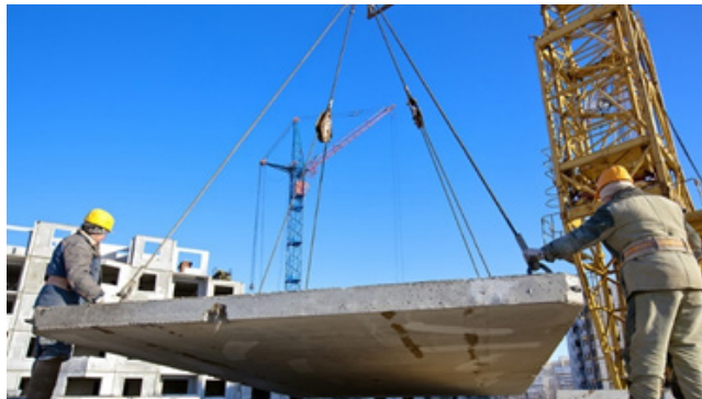
Fig. 1.1.17 Rigging work at site
