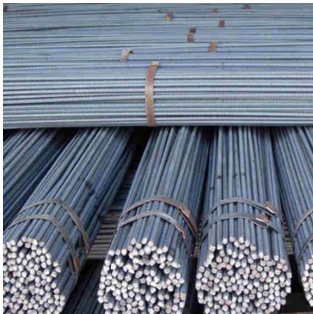
Fig. 4.1.7 Safe and organized storage of cut reinforcement bars
