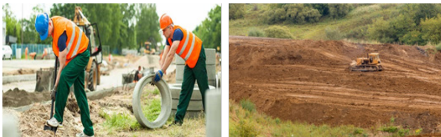
Fig. 9.1.5 Clearing the construction area
