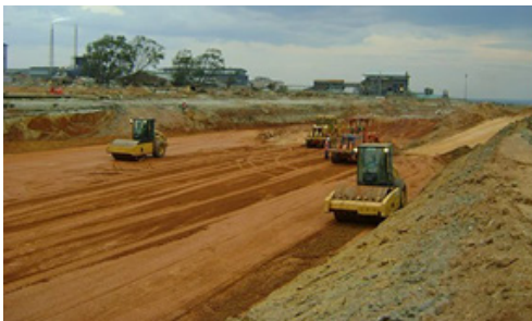
Fig. 9.1.3 Earth work for roads
