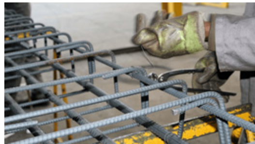
Fig. 1.2.1 Bar bending & steel fixing
