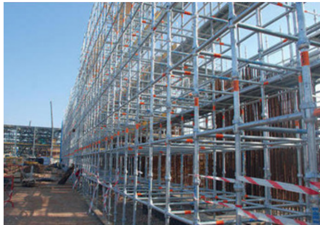
Fig. 6.3.1 Modular scaffolding system
