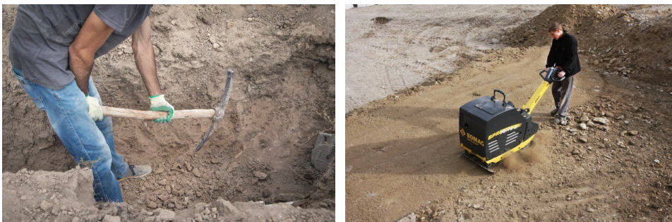
Fig. 1.2.6 Carrying out manual earthwork
