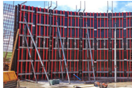
Fig. 1.1.14 System formwork
