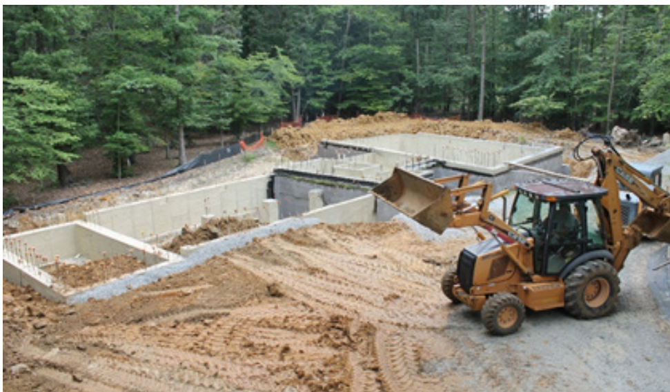
Fig. 9.2.1 Backfilling
