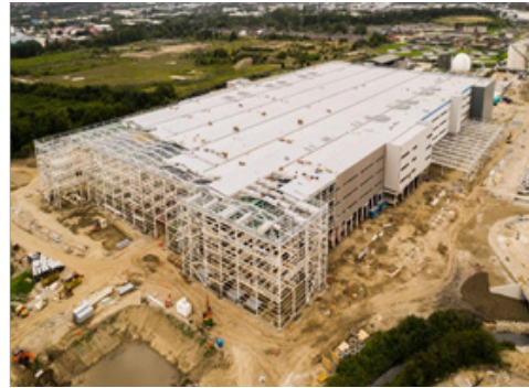
Fig. 1.1.5 Industrial Building Construction Site
