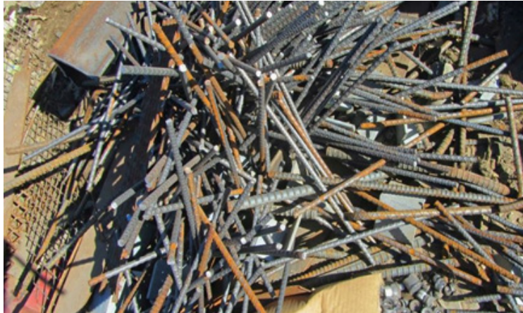
Fig. 4.1.8 Control wastage of reinforcement bars
