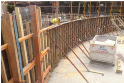
Fig. 1.1.13 Conventional formwork
