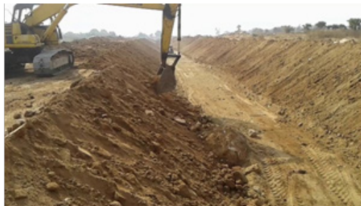
Fig. 9.1.4 Earth work for canals
