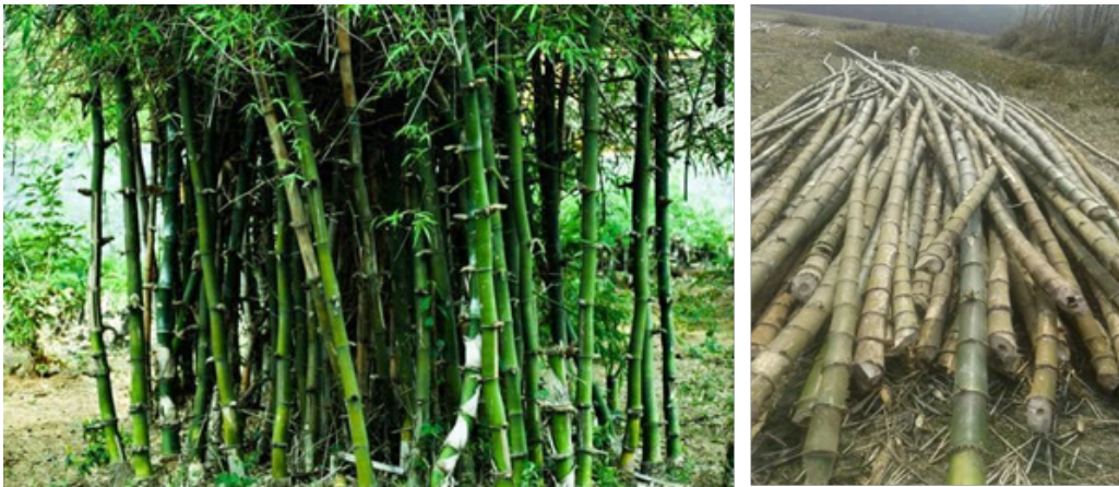
Fig. 6.2.3 Bamboo and ropes used in conventional bamboo scaffolding
