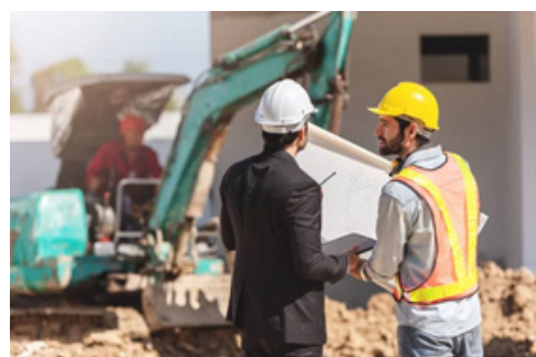
Fig. 9.1.10 Preparatory work prior to earthwork process
