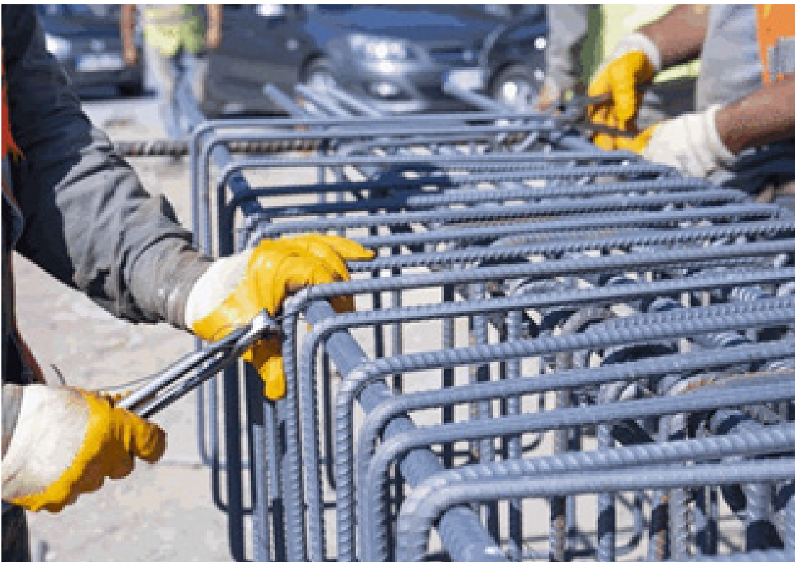
Fig. 3.3.4 Tying rebars for construction use
