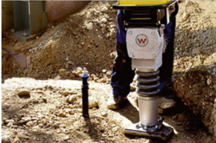
Fig. 9.2.3 Soil compaction by power rammer
