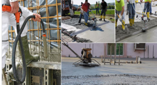
Fig. 9.2.4 Concrete compaction by vibrator
