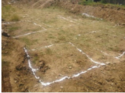
Fig. 9.1.6 Soil marking
