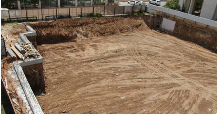
Fig. 9.1.11 Cutting soil manually
