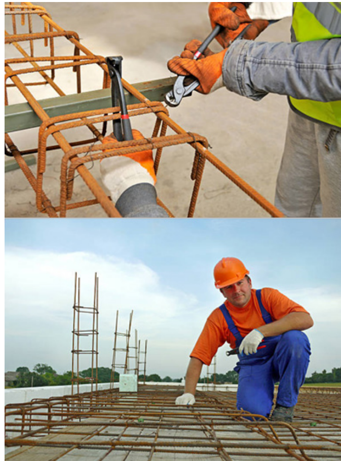
Fig. 1.2.9 A helper bar bender & steel fixer performing his work
