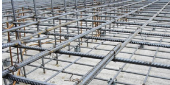
Fig. 1.1.12 Reinforcement bars fixed at site
