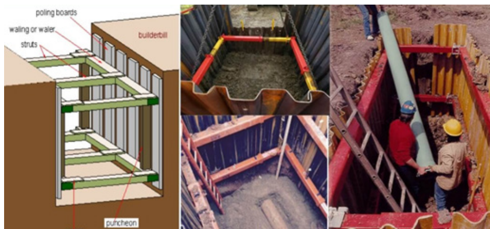
Fig. 9.1.13 Shoring and timbering
