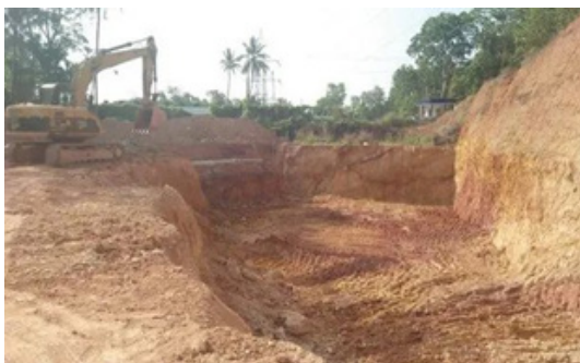
Fig. 9.1.1 Soil excavation
