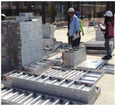
Fig 9.6.3: Stacking of steel panels
