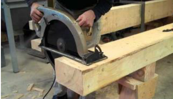
Fig 3.5.7: Cutting board by circular saw
