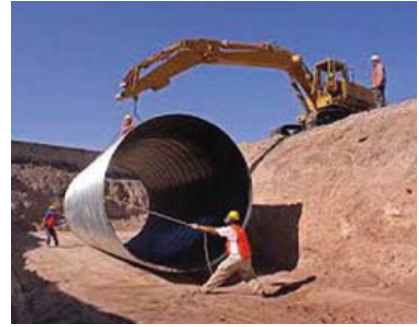
Fig 1.2.9: Rigging work at site
