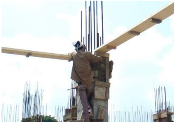
Fig 9.2.12: Erection of formwork for beam
