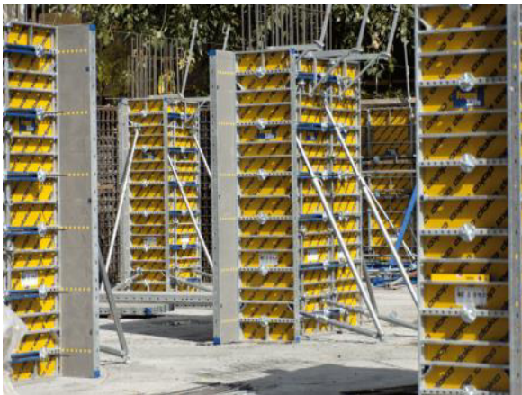
Fig 9.1.13: Doka formwork
