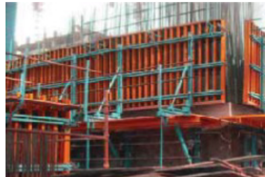
Fig 1.2.6: System formwork
