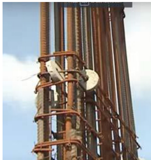
Fig 4.2.7: Checks for Cover blocks
