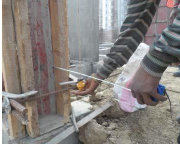
Fig 4.2.5: checks by using Plumb Bob
