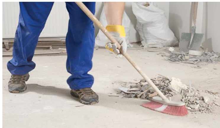
Fig. 7.3.5 Clean-up Debris and Waste
