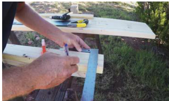
Fig 3.5.6: Measuring and marking on ply board
