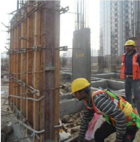
Fig 4.2.4: Checks for verticality
