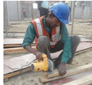
Fig 3.1.21: Use of circular saw
