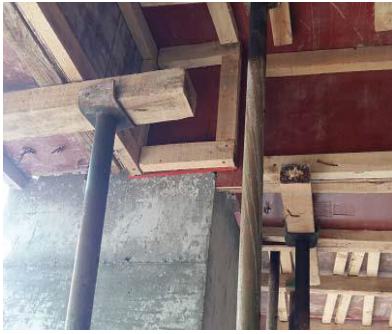
Fig 4.2.16: Checks near the column beam joint 6.5 Fig 4.2.17: props below the panel:
