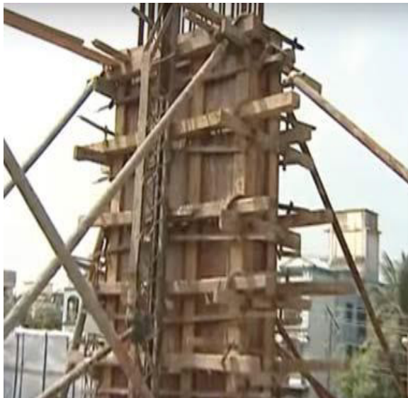
Fig 4.2.6: Checks for props and fixing
