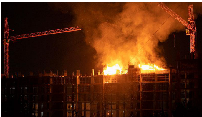
Fig. 7.2.3 Fire at Construction Site
