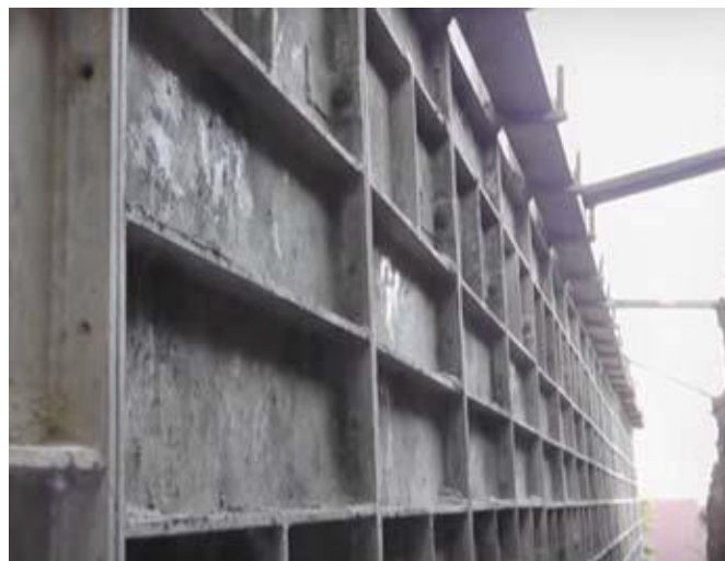
Fig 4.2.10: Wall formwork
