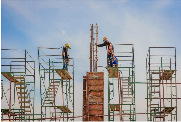
Fig. 5.1.4 Coordination during Construction Work
