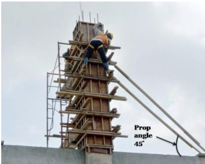
Fig 9.2.8: Fixing props with formwork
