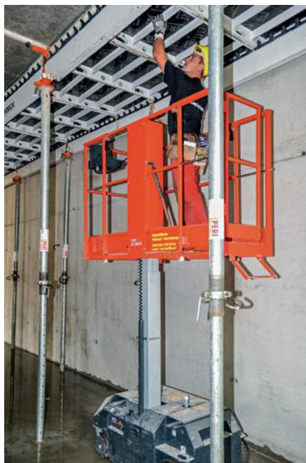
Fig 9.4.2: Stripping components from formwork
