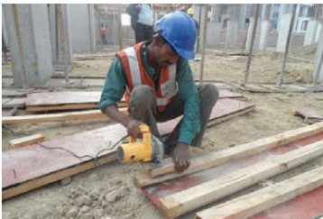
Fig 3.4.20: Cutting wood by circular saw
