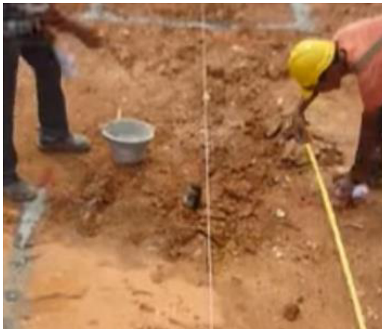
Fig 9.2.1: Measuring and digging footing area
