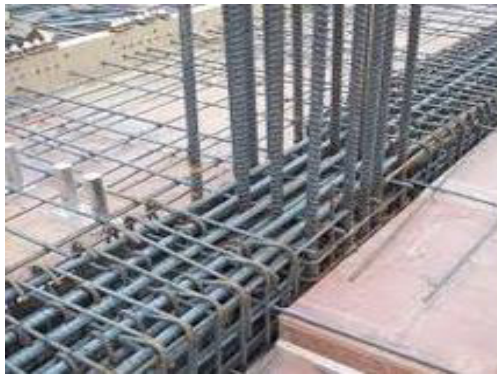
Fig 9.1.32: Construction joint
