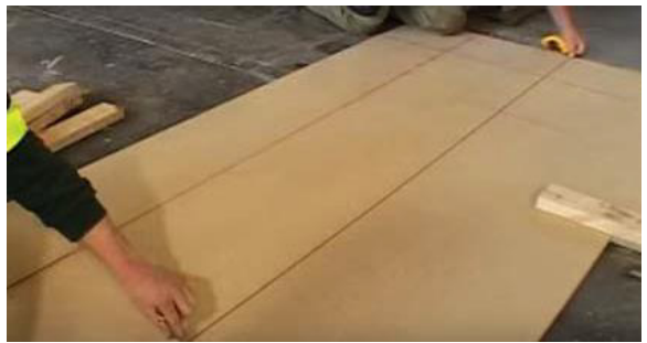
Fig 3.5.9: Measuring wooden board by taperuler
