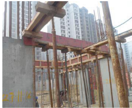
Fig 4.2.15: props below the panel
