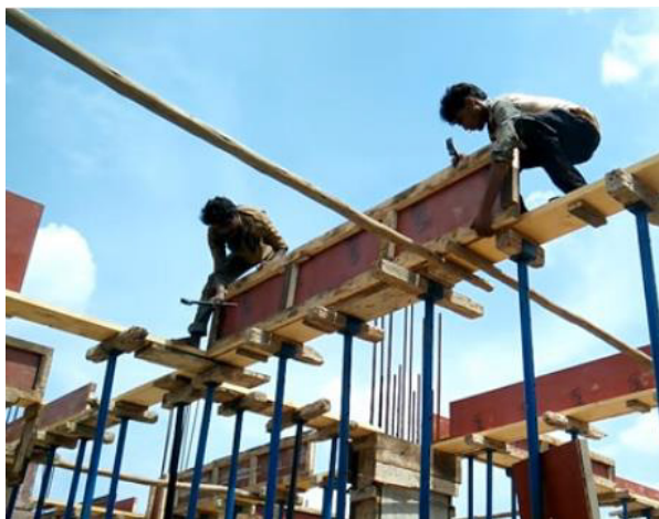
Fig 9.2.13: Fixing of formwork for beam
