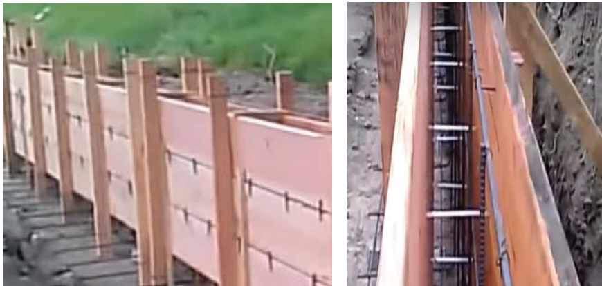
Fig 4.2.8: Wall formwork
