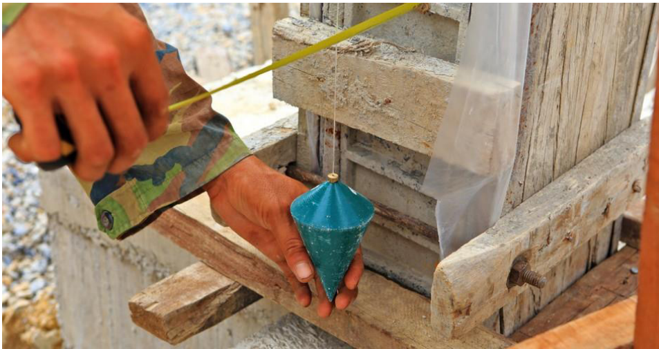
Fig 3.2.3: Use of Plumb bob
