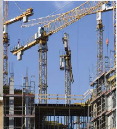
Fig 1.1.4: Industrial Building construction site
