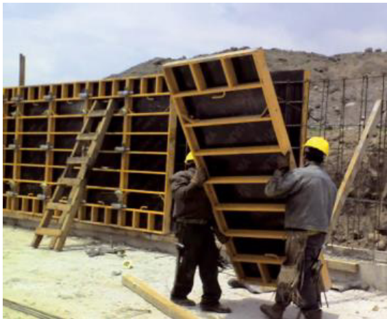
Fig 9.2.21: Dismantling panels from wall
