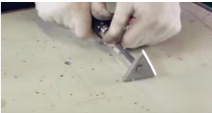
Fig 9.5.3: Cleaning of shutter panel
