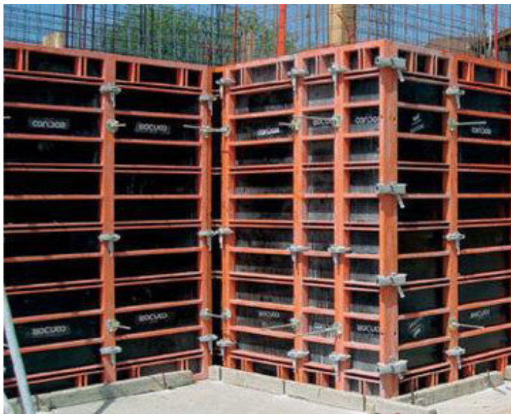
Fig 9.1.12: Steel shuttering
