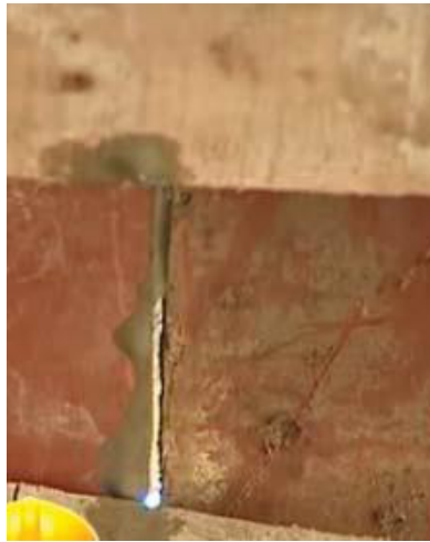
Fig 4.2.13: Checks for damage
