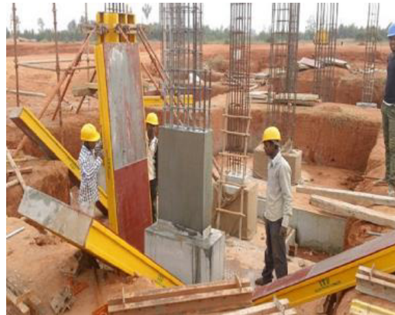
Fig 9.2.22: Dismantling panels from column
