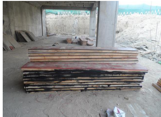
Fig 9.6.2: Stacking of wooden panels
