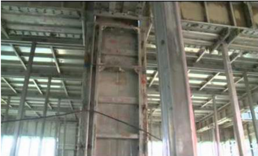
Fig 9.1.11: MIVAN Formwork
