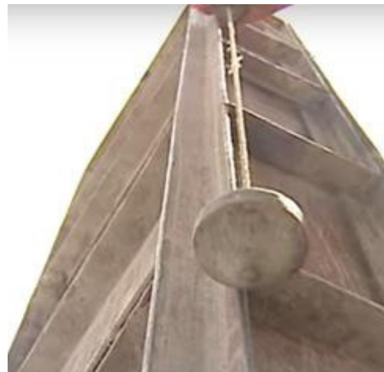
Fig 9.2.7: Checking plumb
