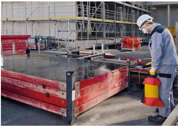
Fig 9.1.30: Application of releasing agents on shuttering panels
