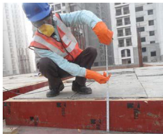
Fig 4.2.12: Checks for dimension of beam and slab formwork
