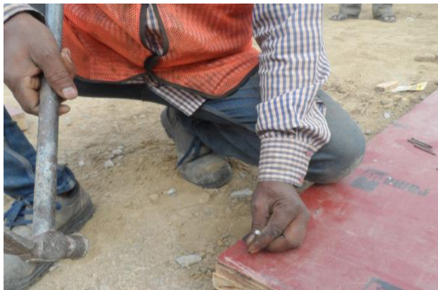
Fig 9.5.1: Repairing by nailing method
