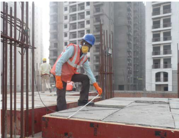
Fig 4.2.12: Checks for dimension of beam and slab formwork
