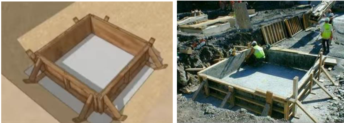
Fig 9.2.3: Erection of formwork for footing
