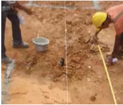
Fig 4.2.1: Measuring footing area
