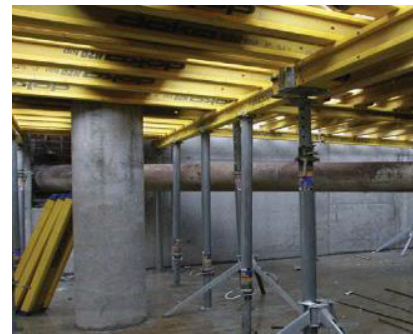
Fig 4.2.16: Checks near the column beam joint 6.5 Fig 4.2.17: props below the panel:
