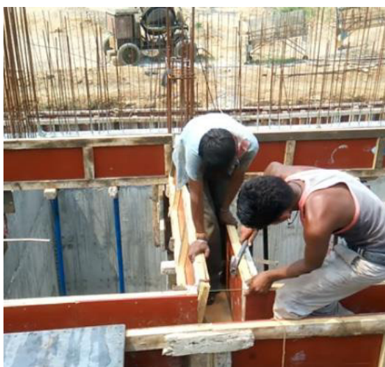
Fig 9.2.14: Fixing formwork for beam
