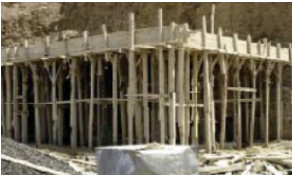
Fig 1.2.5: Conventional formwork
