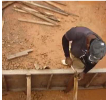
Fig 4.2.2: Fixing footing box
