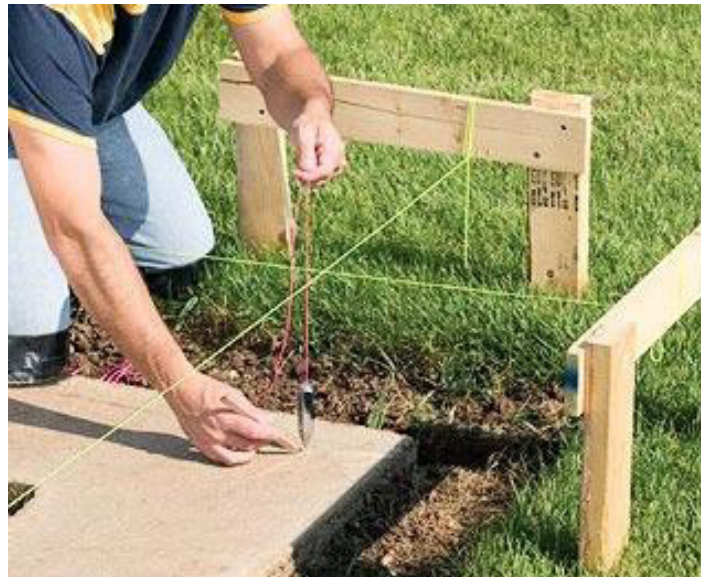
Fig 9.2.4: Centering footing form box
