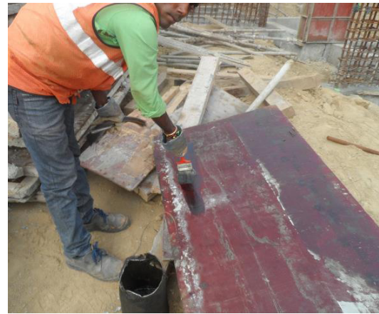
Fig 9.1.30: Application of releasing agents on shuttering panels
