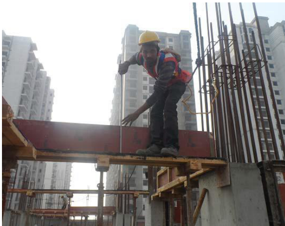
Fig 4.2.14: Measuring depth of panel
