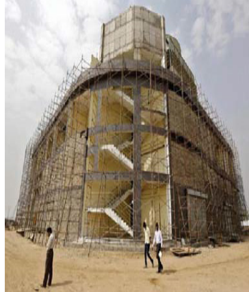
Fig 1.1.3: Building construction site
