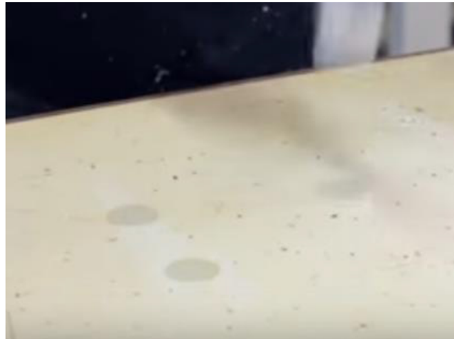
Fig 9.5.8: After repairing by wooden disc
