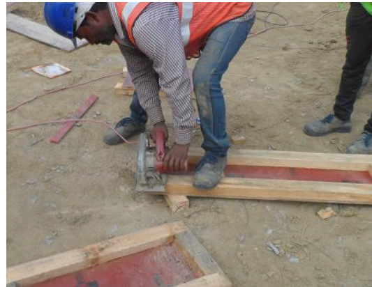
Fig 9.5.2: After repairing by nailing method
