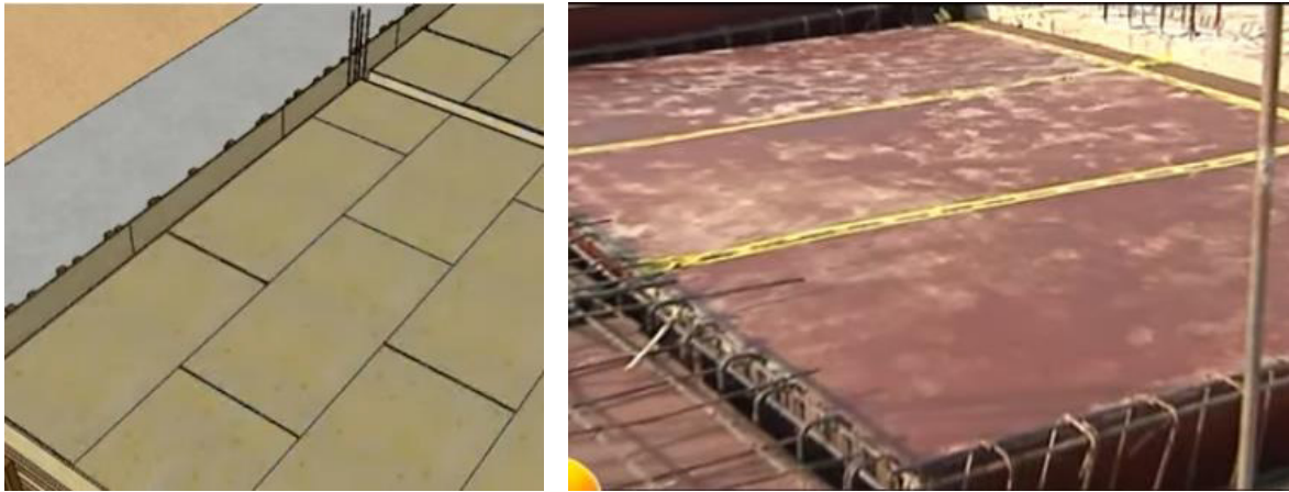
Fig: 9.2.19: Slab formwork
