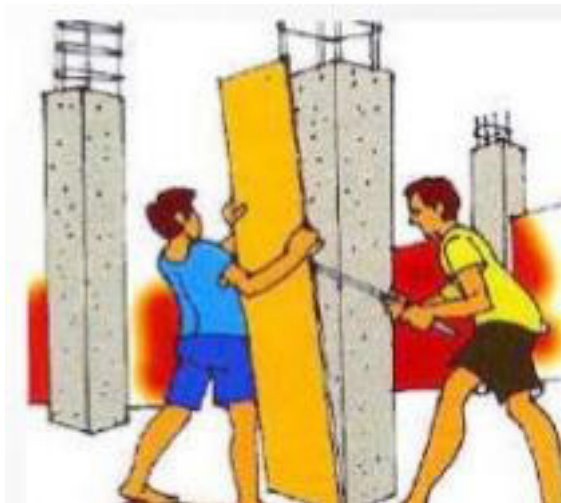
Fig 9.2.20: Dismantling of column formwork
