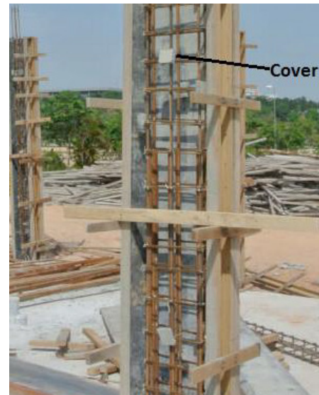
Fig 9.2.9: Cover in column formwork
