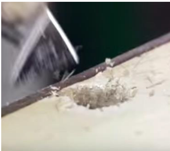
Fig 9.5.9: Filling corners by wood filler
