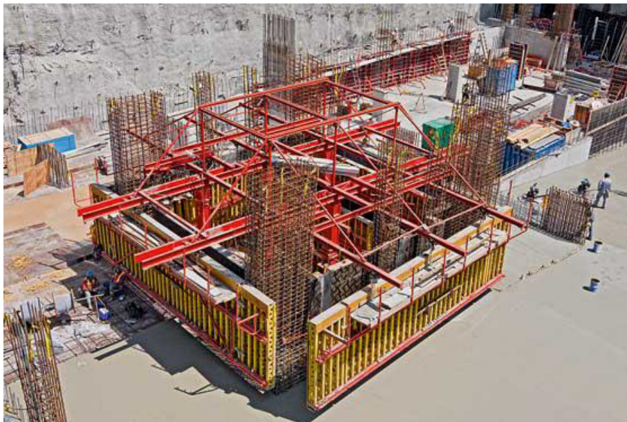
Fig 9.1.20: Peri formwork
