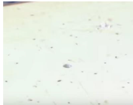
Fig 9.5.4: Shutter panels after removing Paint
