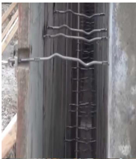
Fig 4.2.9: Wall formwork
